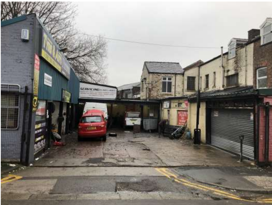
Image 6 – View to rear elevation and service yard
