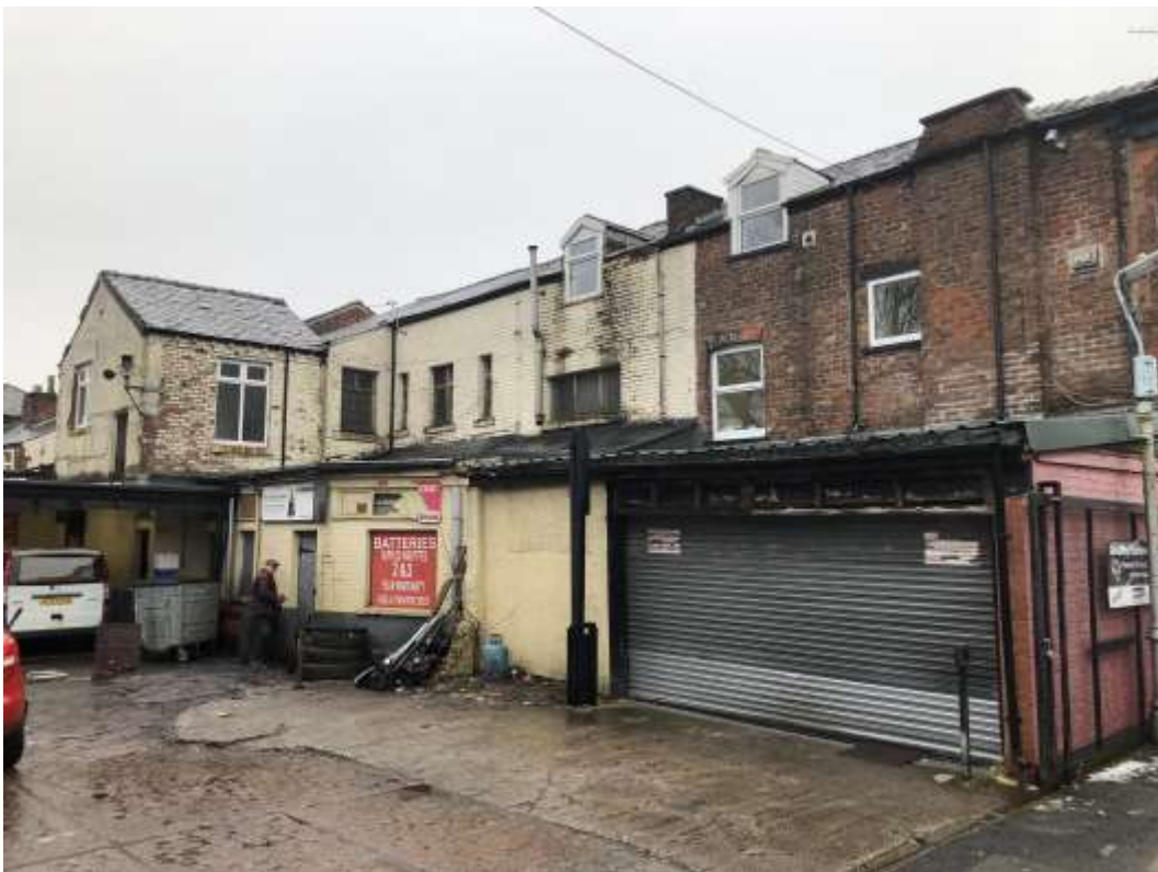
Image 8 – View to rear elevation & service yard
