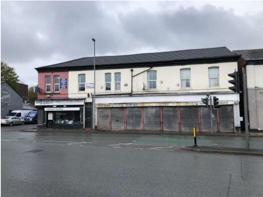
Image 5 – View to front elevation and gable elevation of Northern Crafthouse
