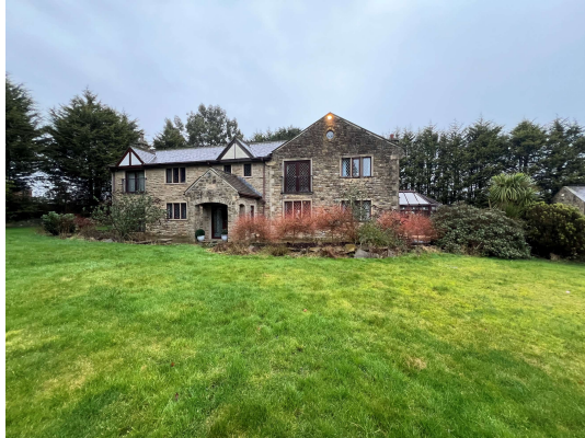
View of the front façade of the existing dwelling
