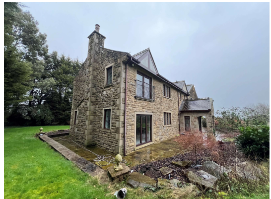
View of the side (north) façade of the existing dwelling
