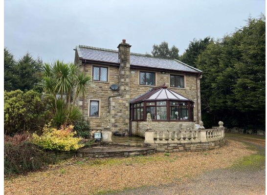
View of the side (south) façade of the existing dwelling
