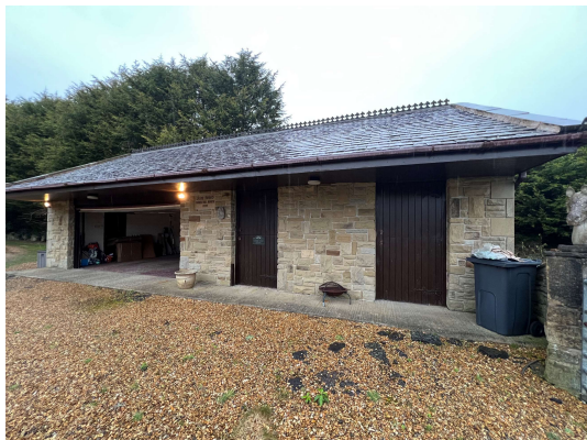
View of the existing detached garage
