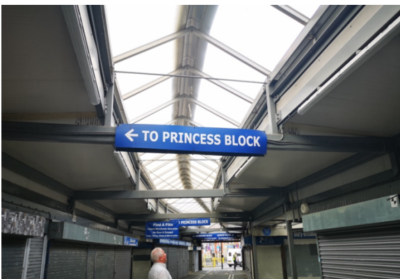
Typical Existing Canopy
