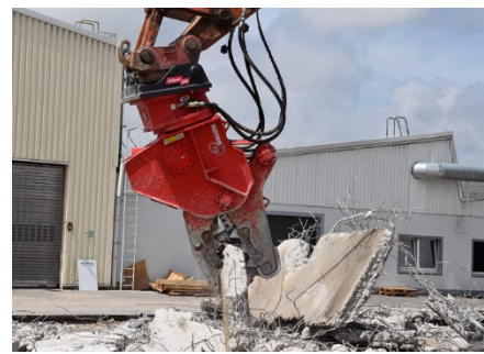
Machine mounted pulverising jaw
