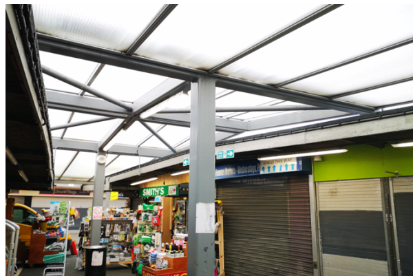
Typical Existing Canopy
