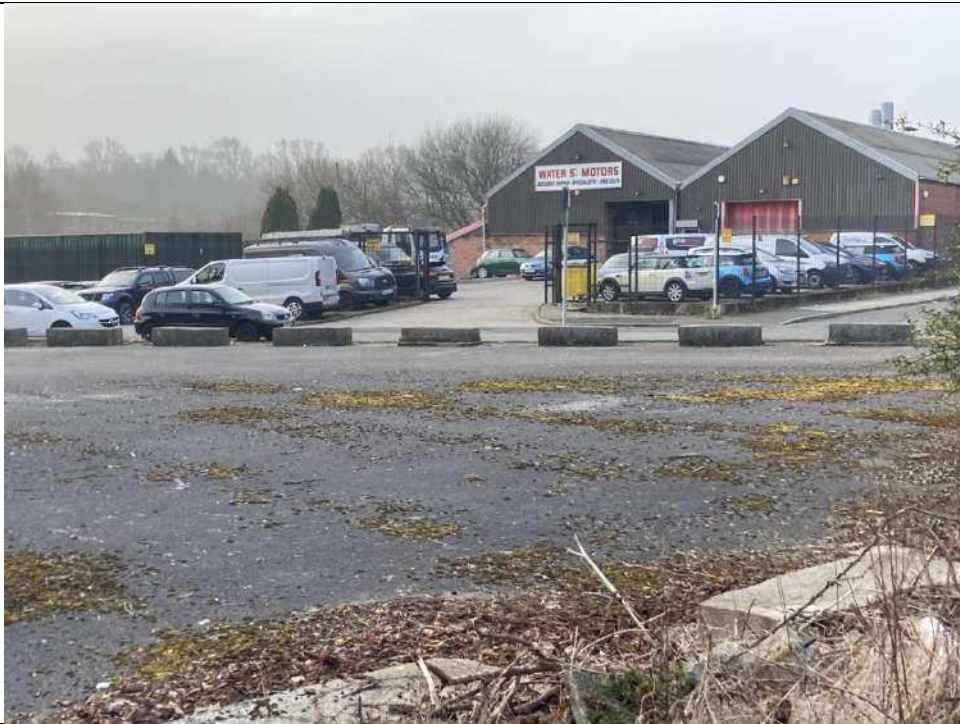
Plate 27 – Garage works south west of site
