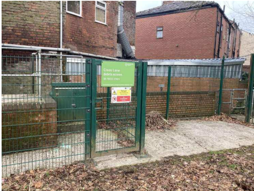
Plate 25 – Cross Lane debris screen, north of site
