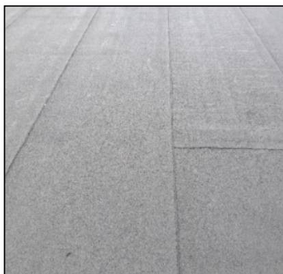
Flat roof construction with a bitumen felt finish.
