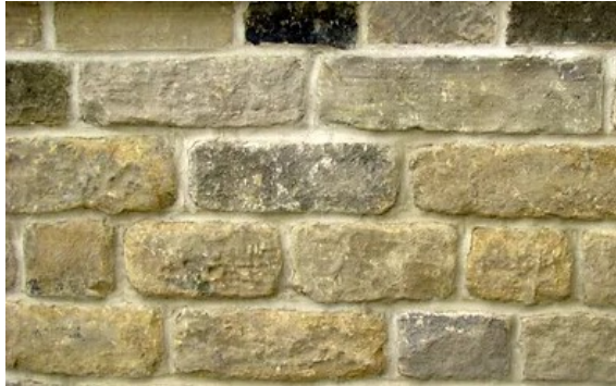
Locally sourced Sandstone to match existing finish.
