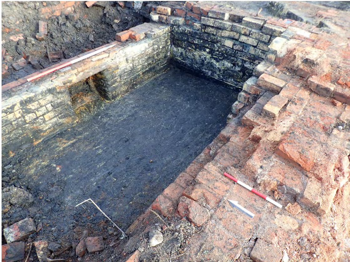
Fig. 4.9: View looking NE across the east end of economiser chamber 117
