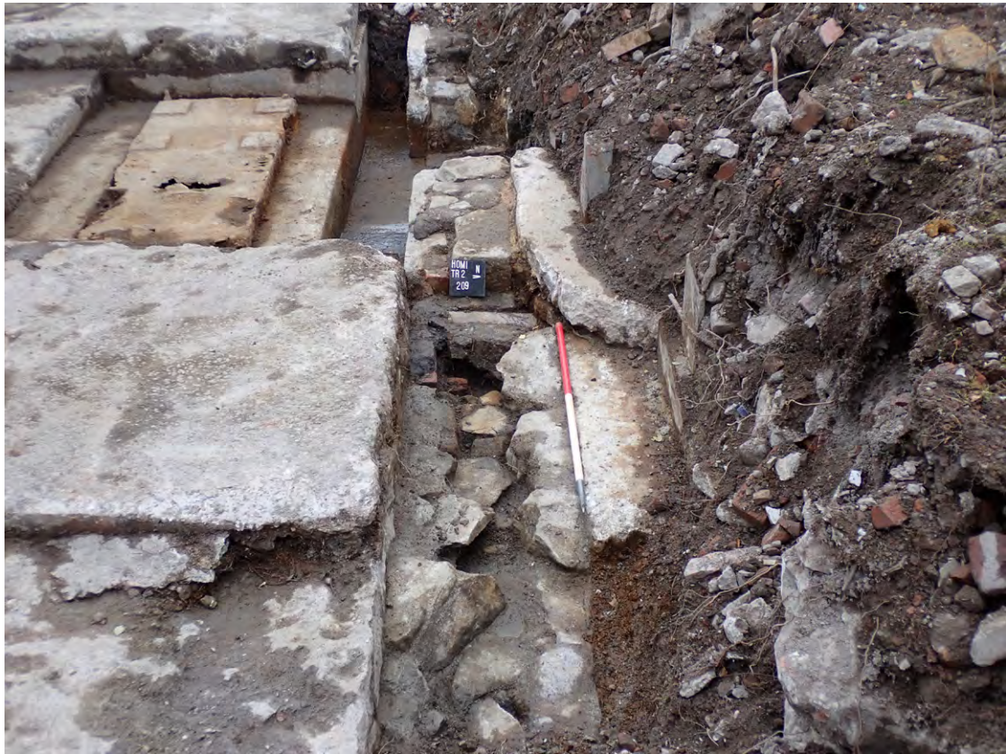
Fig. 4.15: View looking west along foundation 209
