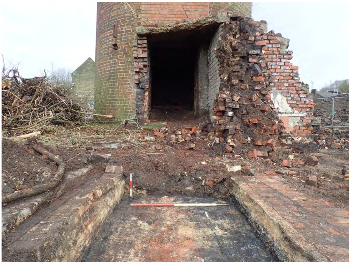
Fig. 4.13: View looking north along main flue towards the chimney stack
