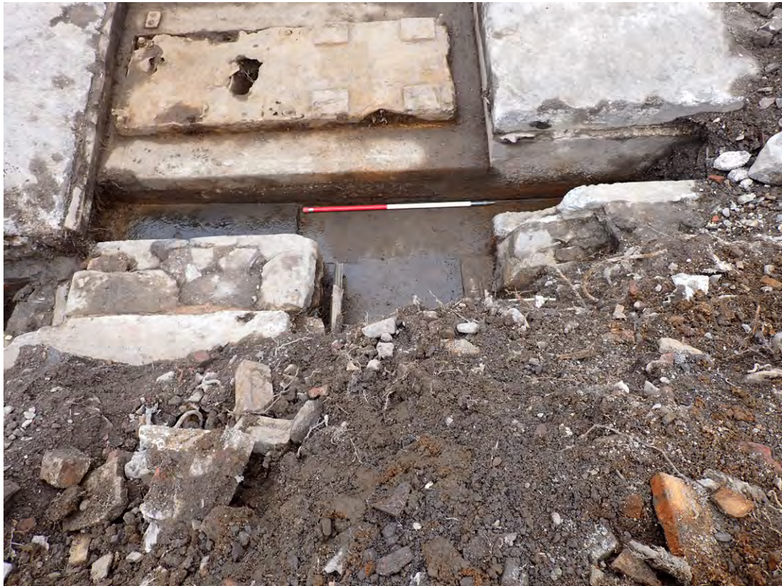
Fig. 4.17: View looking south at culvert 210
