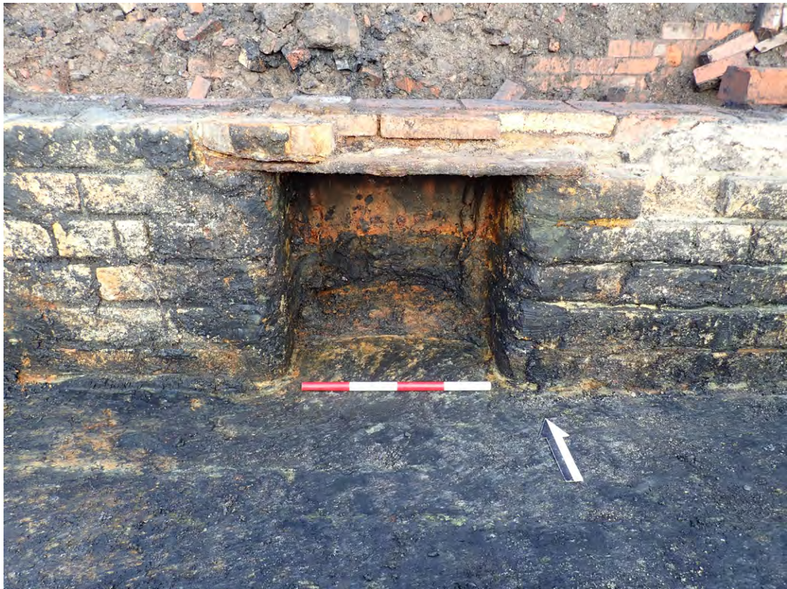
Fig. 4.10: Access hatch in south facing internal elevation of economiser chamber
