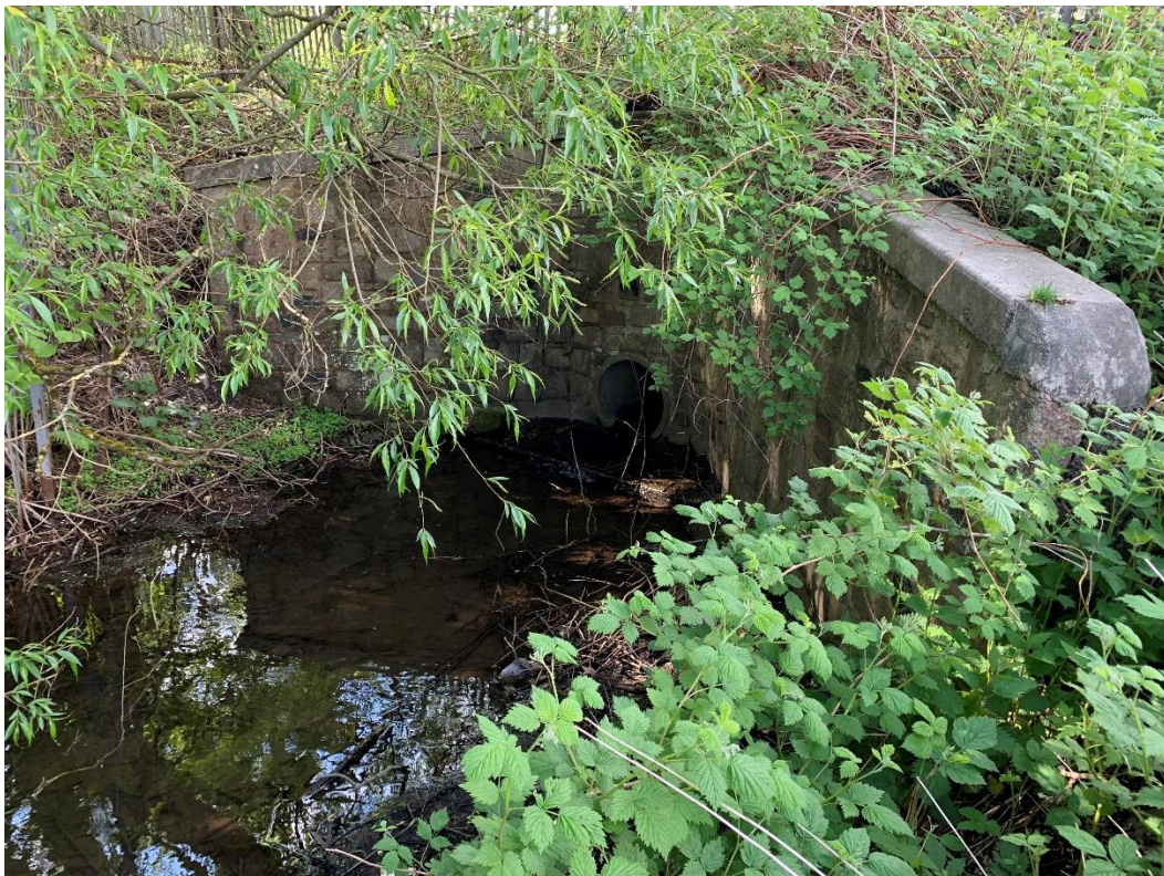
6 – Pipe Outlet to stream
