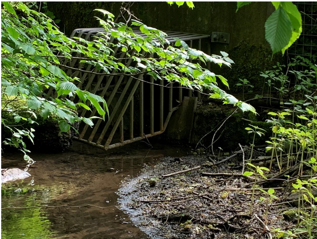
12 – Grill to pipe inlet beneath railway embankment
