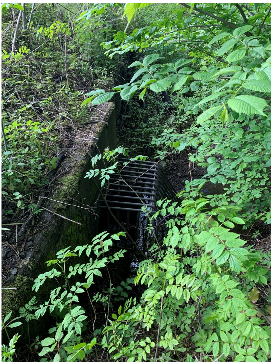
13 – Grill to pipe inlet beneath railway embankment
