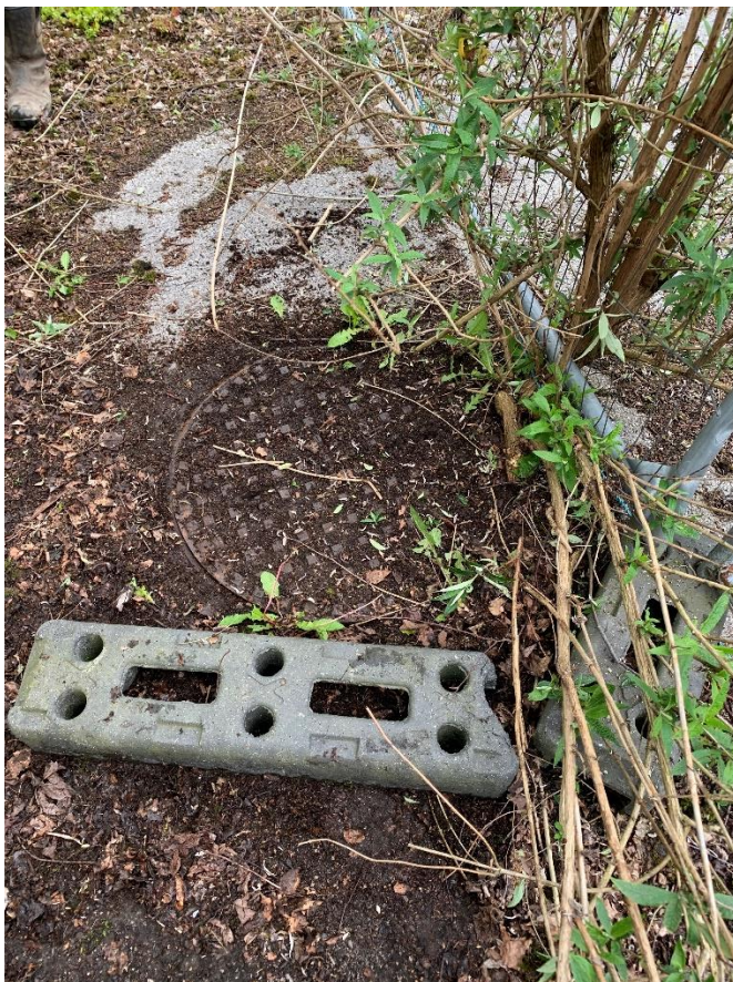
2 – MH on pipe
