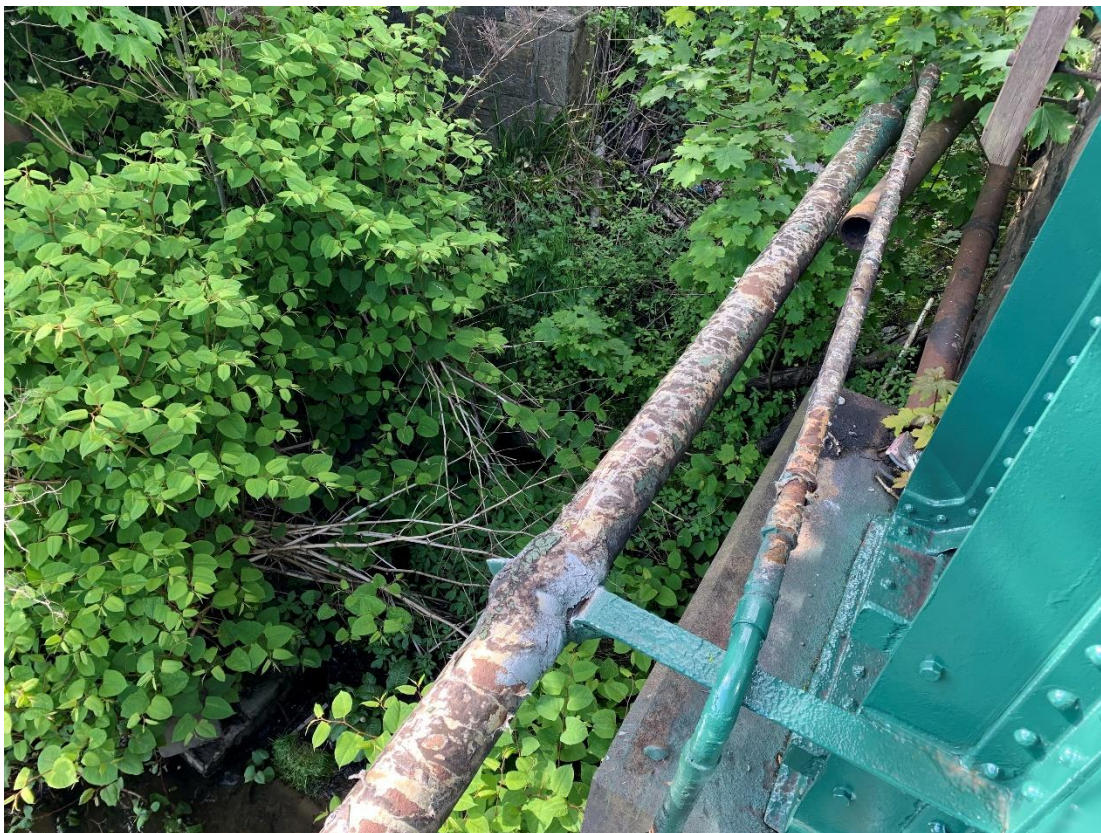
17 – Outfall to River Irwell
