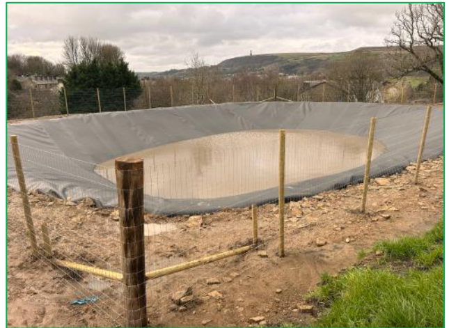
The newly installed slurry pit
