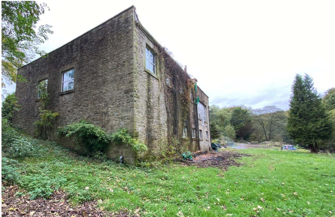
East side of building showing garden falling to the river bank on the right hand side.
