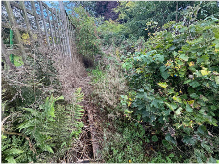
Looking west at south end
