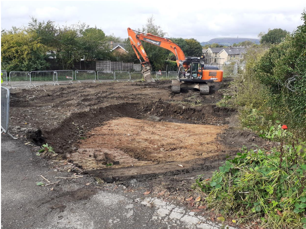
Pic 4 – JK area completed
