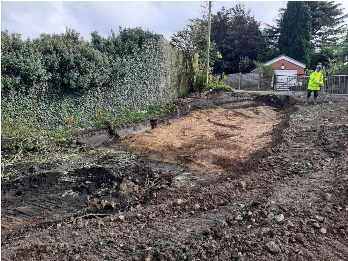
Pic 3 – Jk area Excavated
