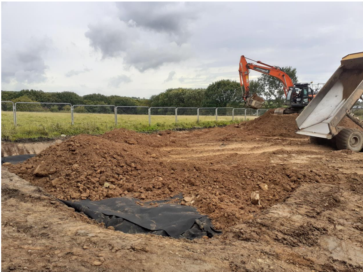
Pic 6 – Burial cell covered in clean soil prior to completion of finished surface levels (+ 1.0m minimum)
