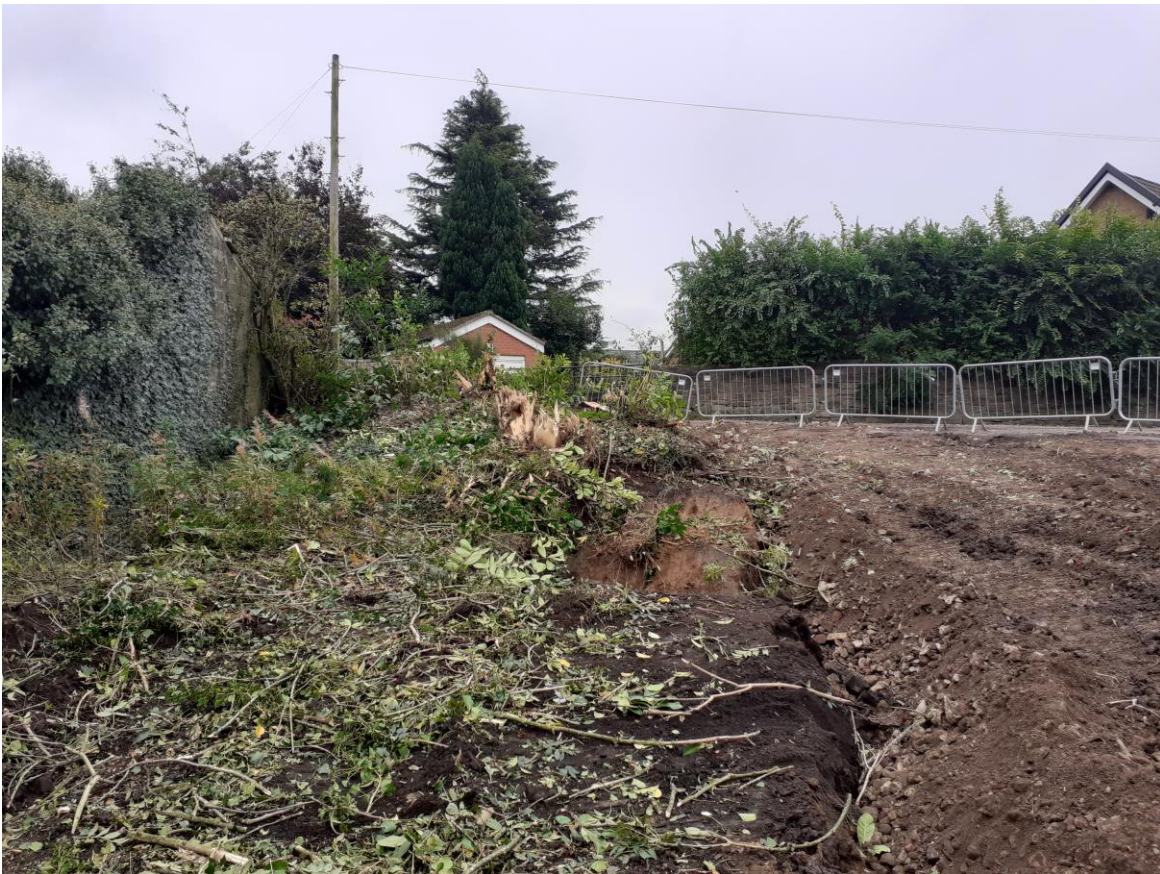
Pic 2 – JK area during excavation
