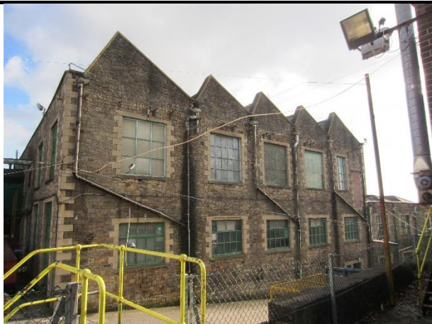
Photo 19: West elevation of Building 7
