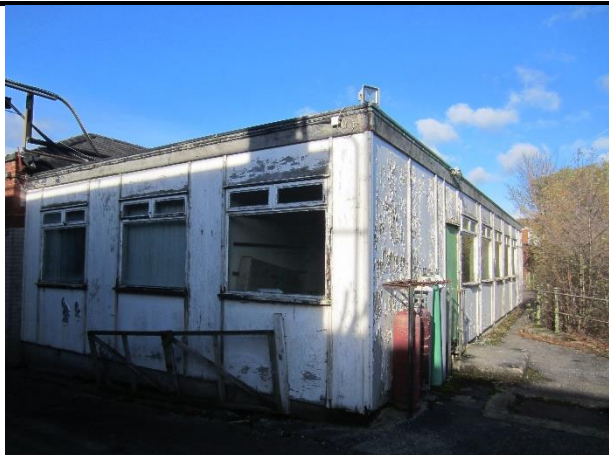
Photo 13: Building 4b, portacabin attached to the east elevation of Building 3
