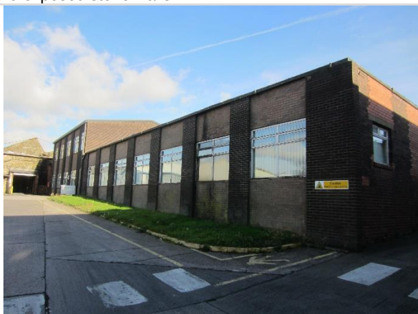
Photo 9: West and south elevation of Building 4
