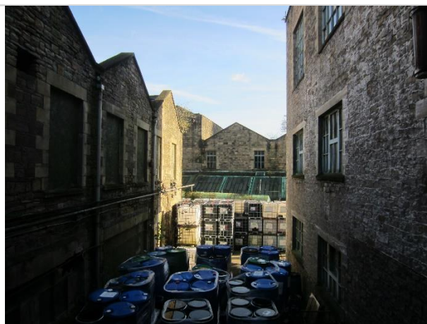
Photo 16: Buildings 5b (left) and 7 (right)
