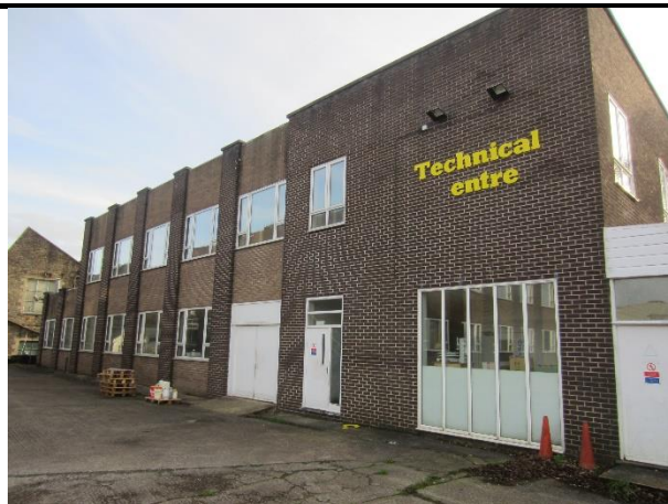
Photo 26: North and west elevation of Building 10
