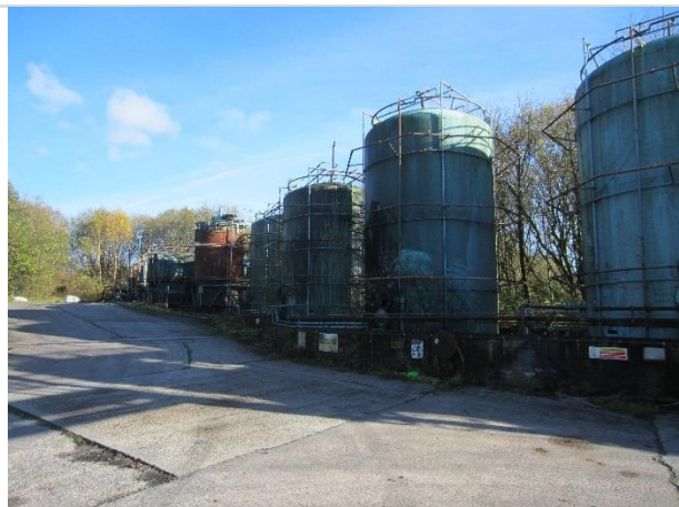
Photo 9: Hard-standing around the operational Tetrosyl site
