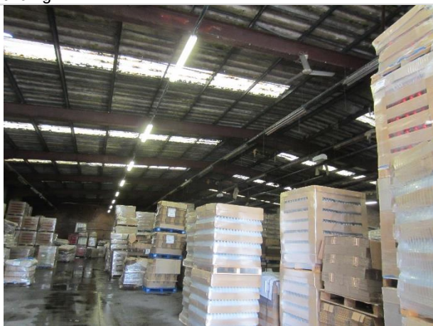
Photo 23: Interior of Building 8
