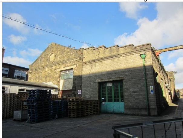
Photo 28: South elevation of Building 11c (11d to the left)
