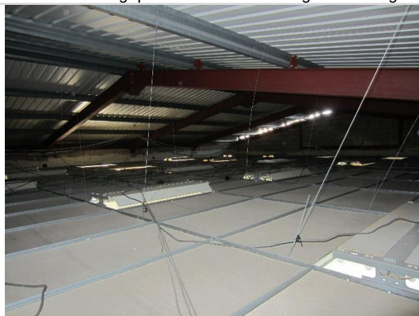
Photo 12: Roof void above suspended ceiling at two-storey section of Building 4a
