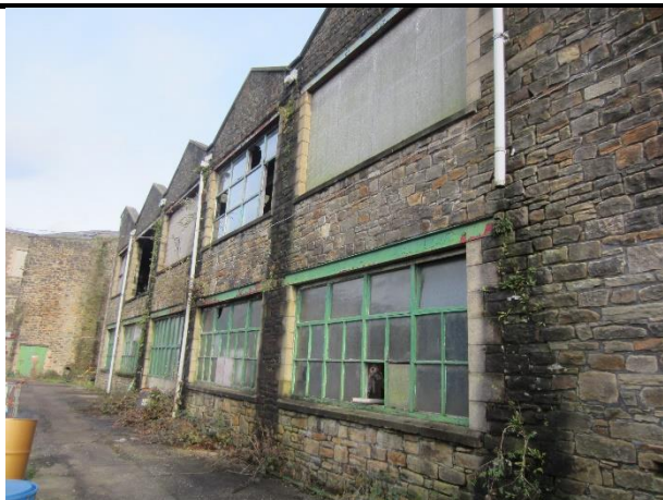
Photo 31: West elevation of Building 13
