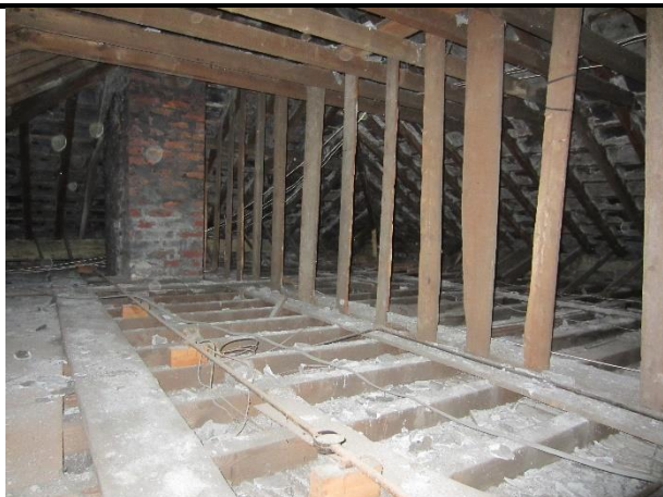
Photo 25: Roof void at Building 9
