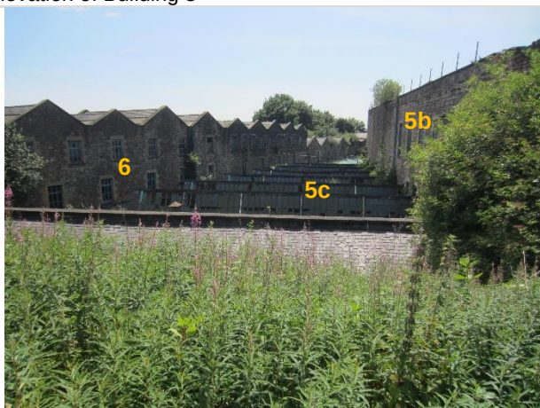
Photo 15: Building 6, 5c and 5b (left to right)
