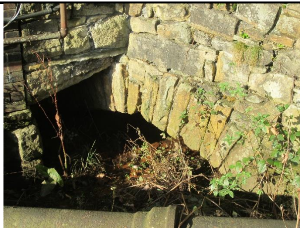
Photo 38: Culvert entrance near weir
