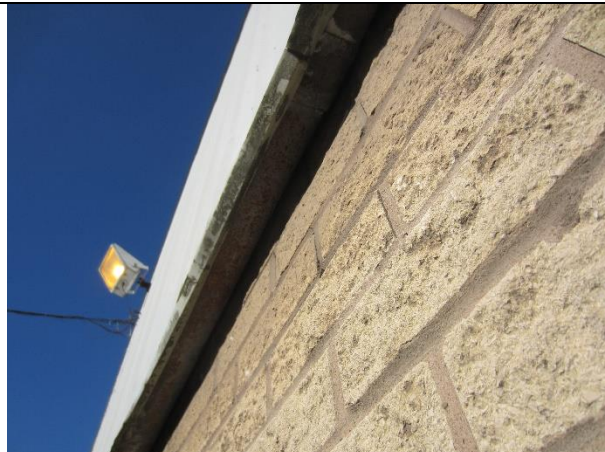
Photo 2: No gaps present beneath the cladding or in the blockwork at Building 1
