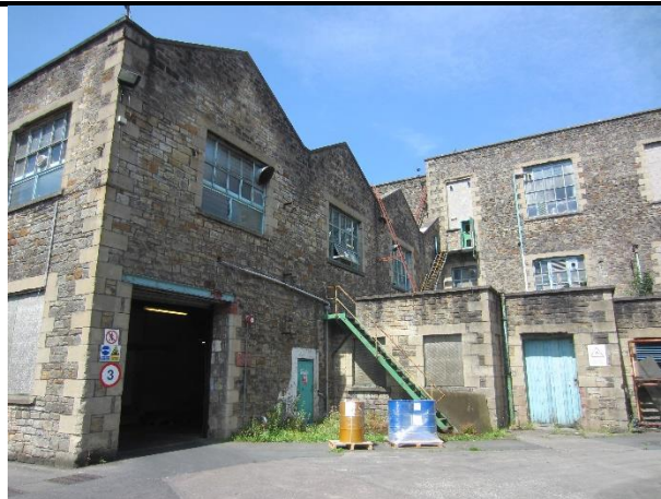
Photo 20: South elevation of Building 7 (5b in background)
