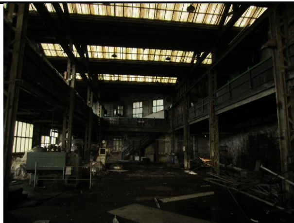
Photo 32: Interior of Building 13
