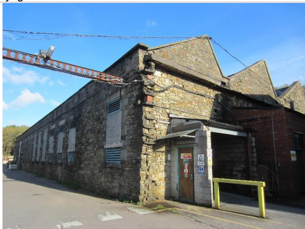
Photo 5: West and south elevation of Building 3
