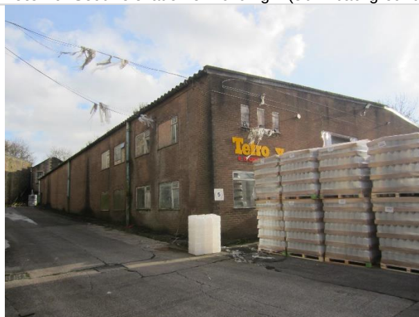
Photo 22: North and west elevation of Building 8
