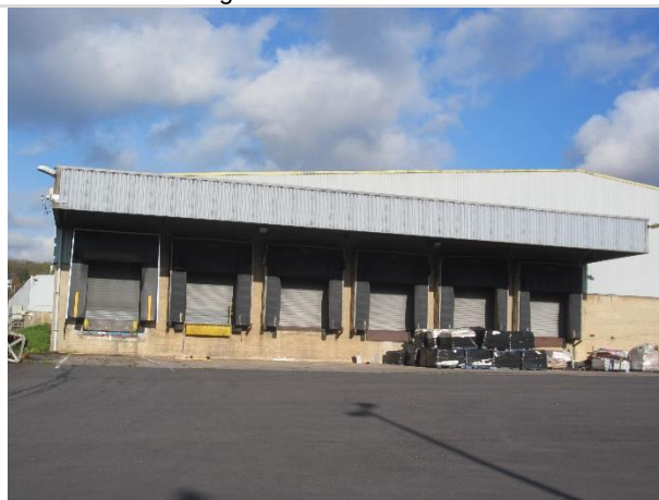
Photo 4: South elevation of Building 2
