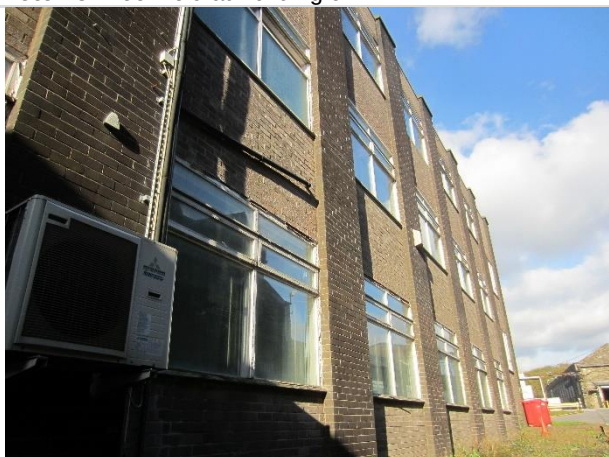
Photo 27: East elevation of Building 11b
