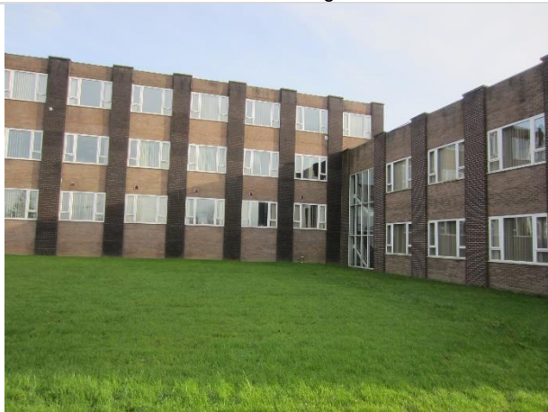
Photo 29: West elevation of Building 11b and north elevation of 11a
