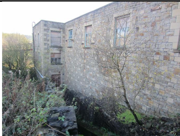
Photo 14: North elevation of Building 5a
