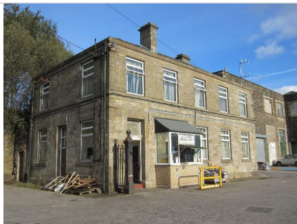
Photo 24: West and south elevation of Building 9
