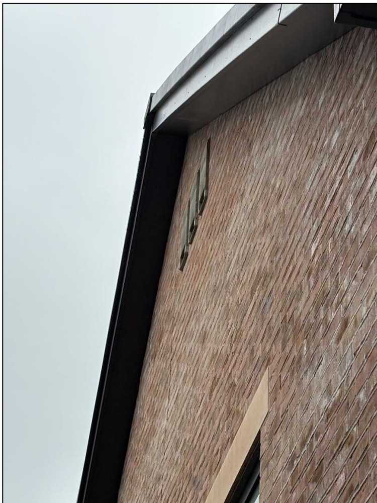
Figure 2. Schwegler Bat Tubes installed at the northeast gable
