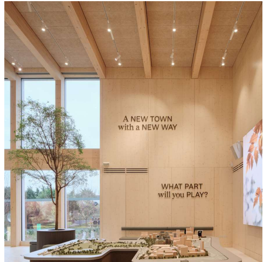
Figure 18 – Timber construction case study: Brent Cross Pavilion, London. Designed by Expedition, a similar timber construction has been used. This has achieved embodied carbon emissions associated with the building structure of 250 kgCO 2 /m 2 , meeting best-practice LETI embodied carbon targets.
