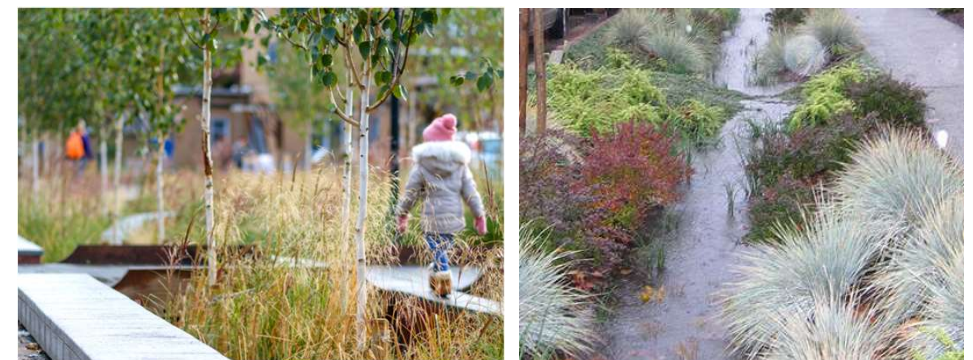
Figure 22: Typical source control SuDS measures
