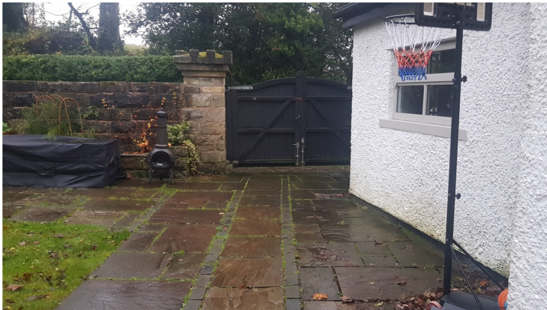
View of gate and wall from inside property
