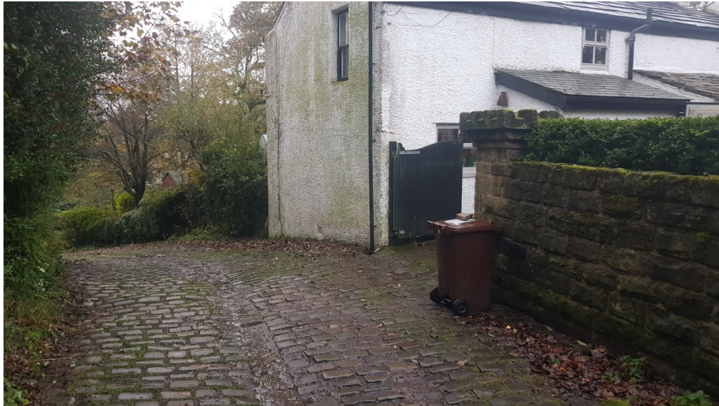
Existing Rear gate and wall
