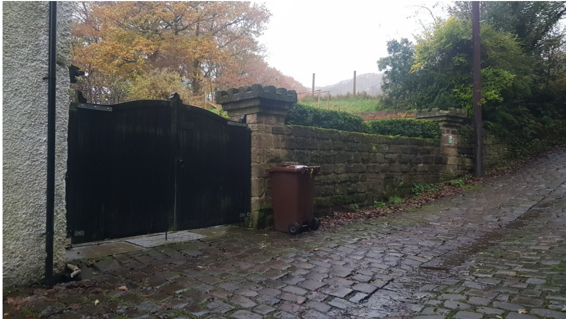
Existing gate and wall. Proposed would mirror this with gate moved north
