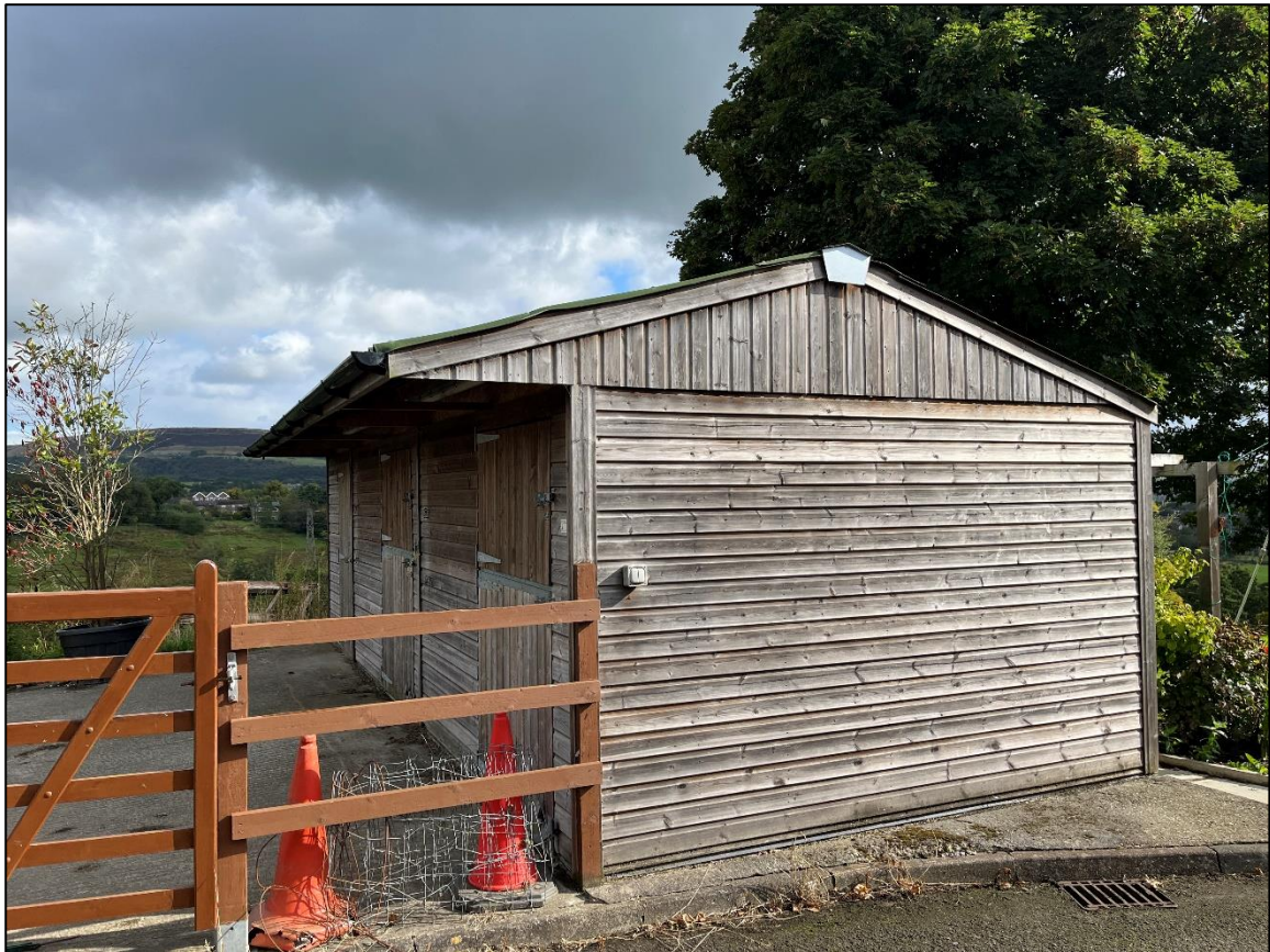
Plate 13 – Further B3 structure
