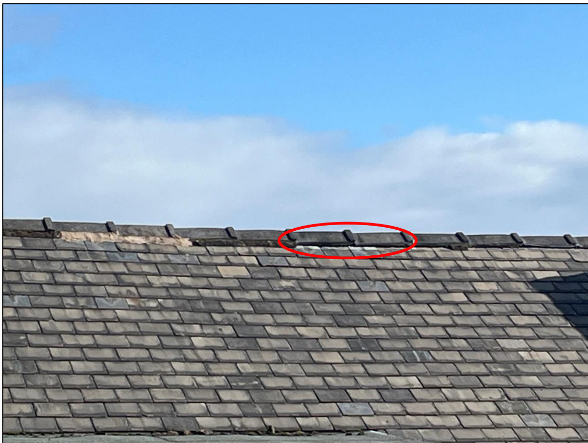
Plate 9 – Example of PRF beneath ridge tiles of B1
