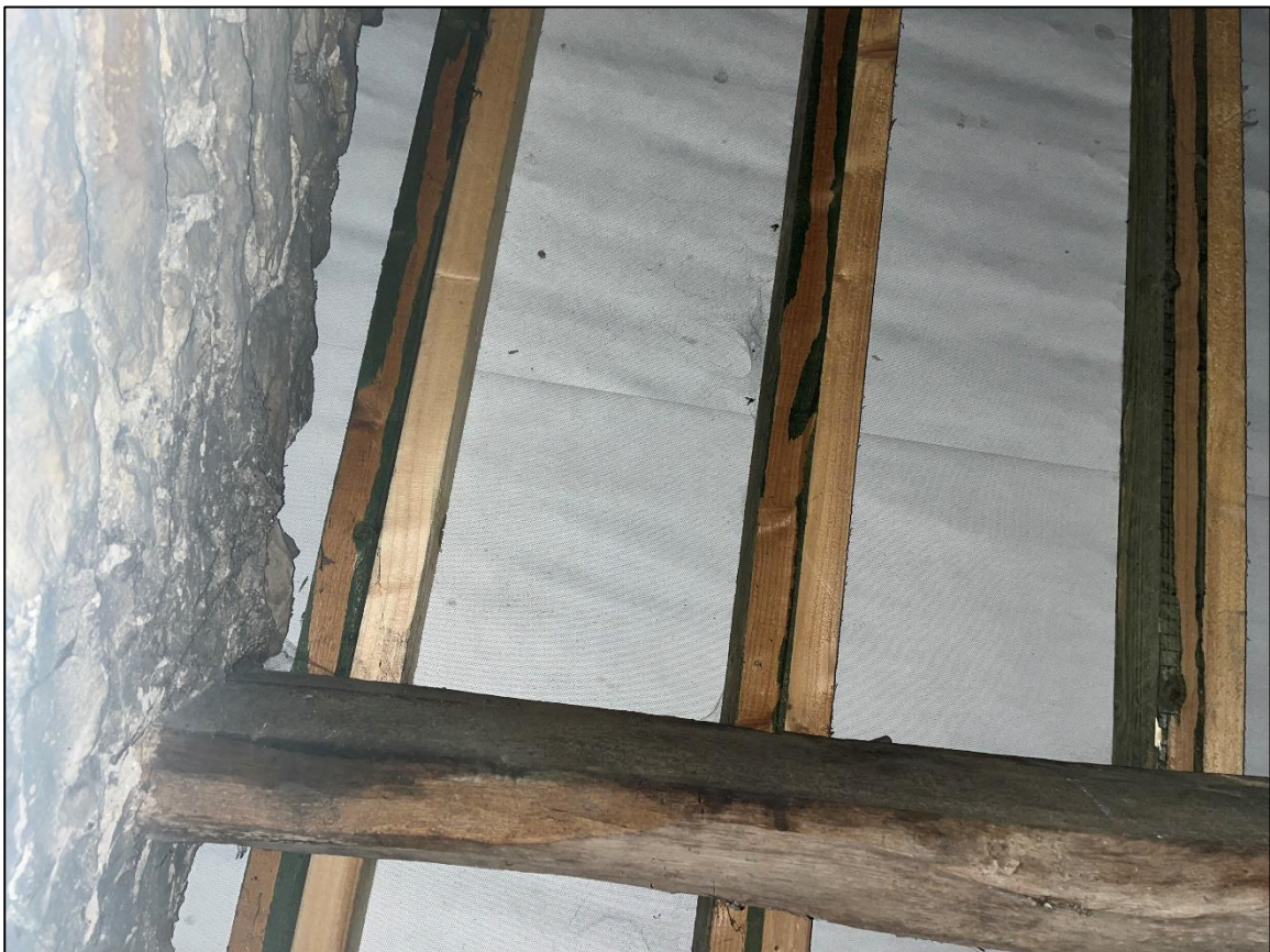
Plate 6 – BRM within loft space
