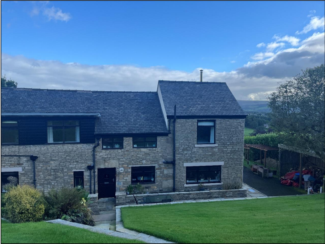
Plate 1 – Southern aspect of dwelling (B1)
