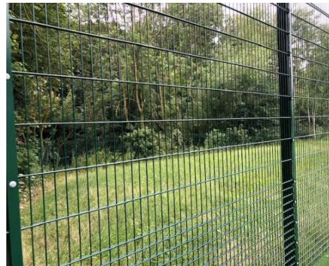
Rigid panel ballstop fencing to perimeter of facility, powder coated dark green so discrete against a rural backdrop
