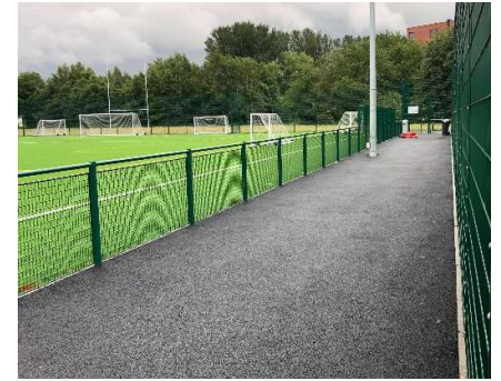
Porous macadam hardstanding to side of pitch
