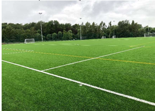
Typical example of 3G artificial turf
