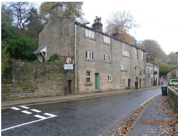
Gable of 26 with entrance and canopy. Shoulder of Mutton/Alba Street on the right.
