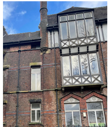
Third Floor bay windows
