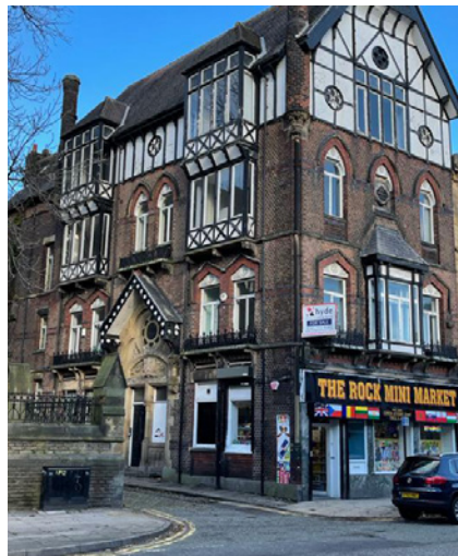
View of two principal façades
