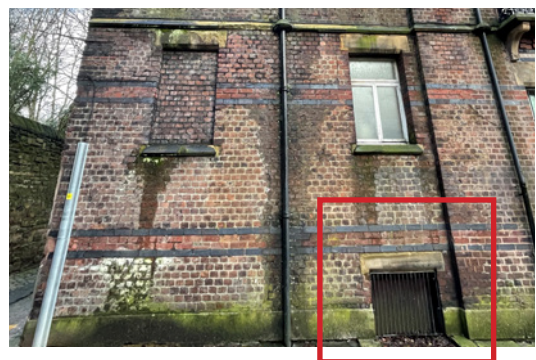
Existing basement windows that are to be reinstated.
