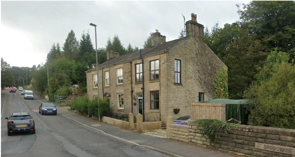
Dwellings on Holcome Rd, south of Holymount Lane entrance
