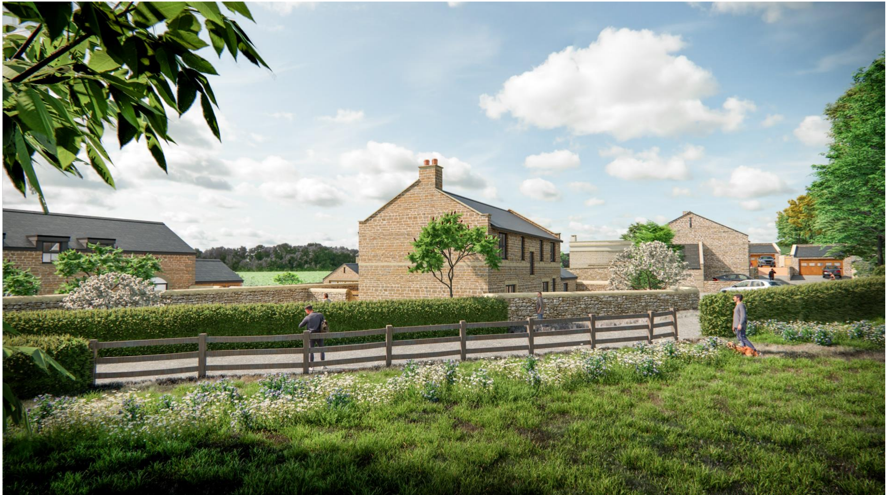
Figure 28. View of Proposed Development from Hollymount Lane pedestrian crossing
