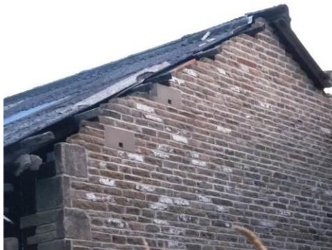
Example of Forticrete boxes in situ
