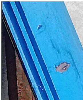
Photograph of existing Inner profile of the front door glazed panel, Proposed work should match to existing
