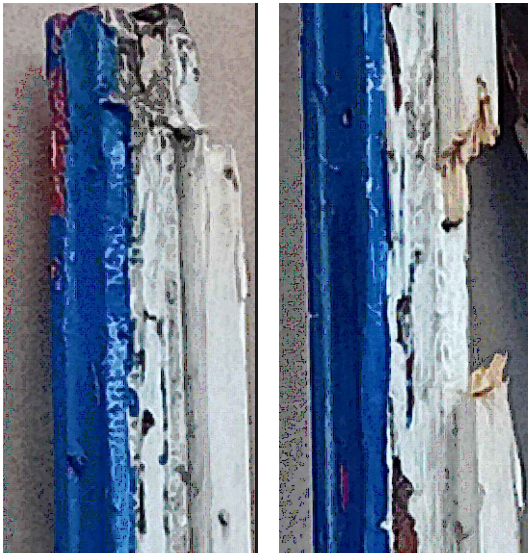
Photographs of existing profiled timber of the shop front, Proposed work should match to existing
