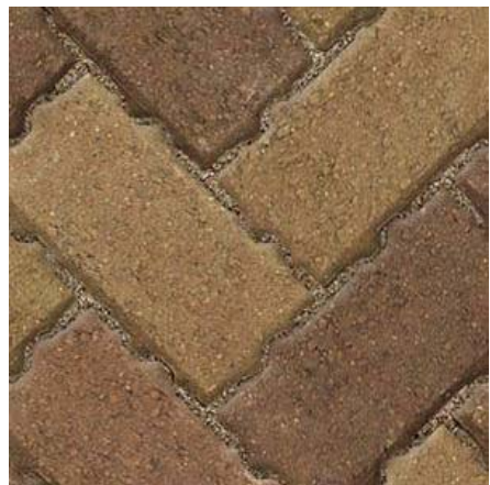
3. Materials - Permeable Block Paving - Yard 1:1
