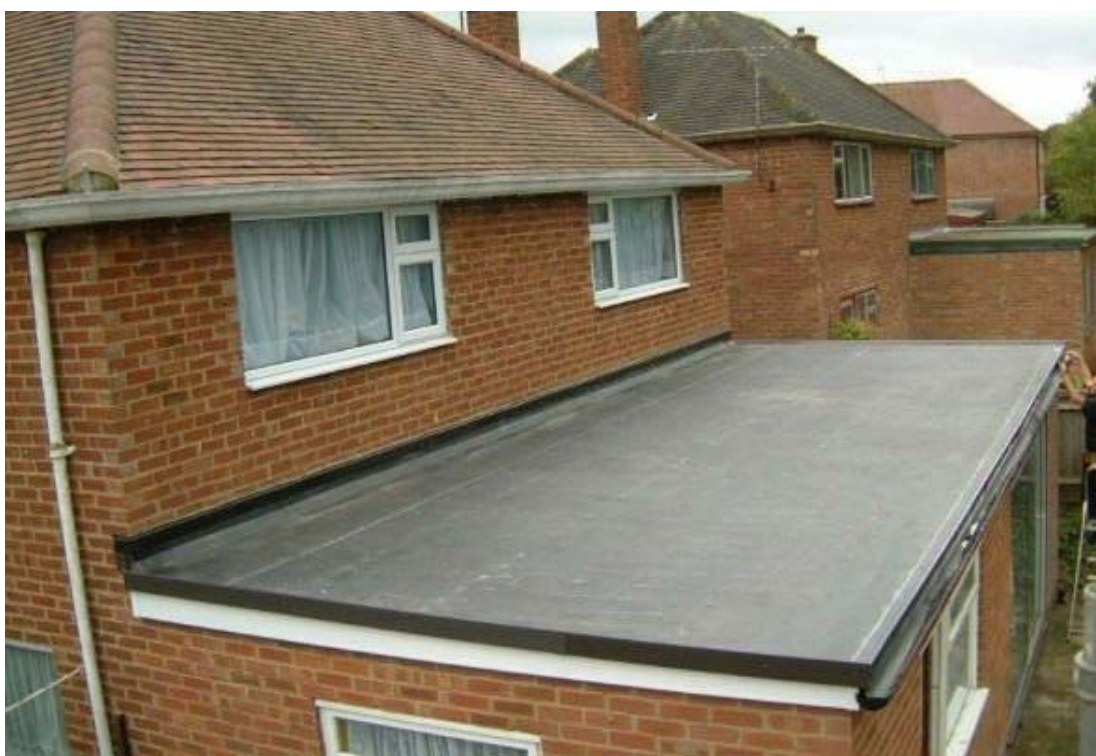
3. Single ply high performance roofing membrane
