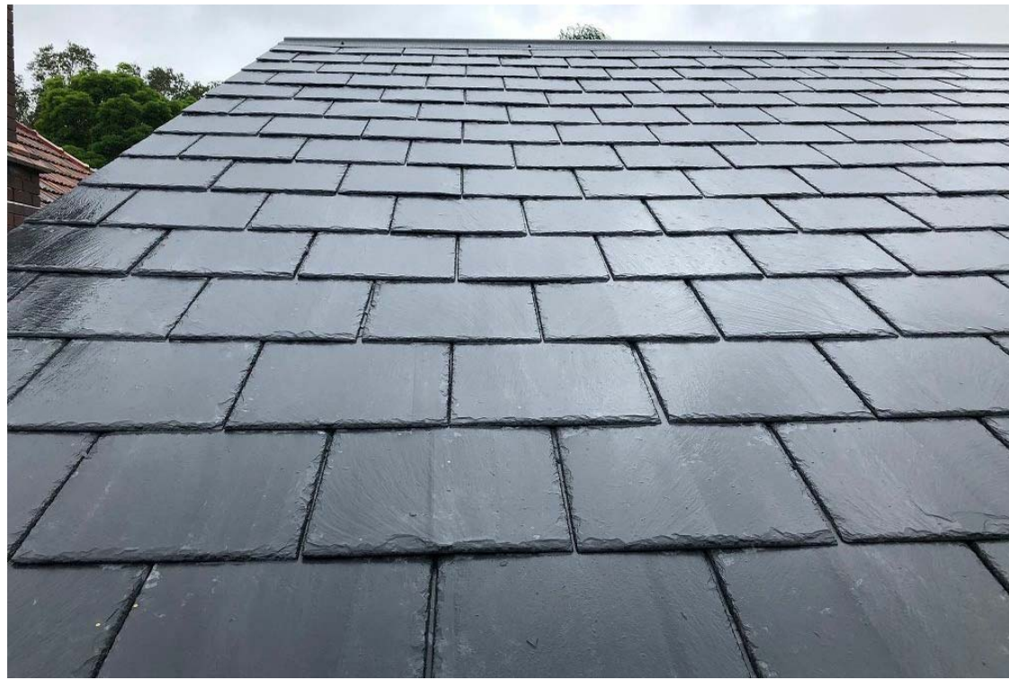
2. Natural Slate Roofing Tiles to Match Existing
