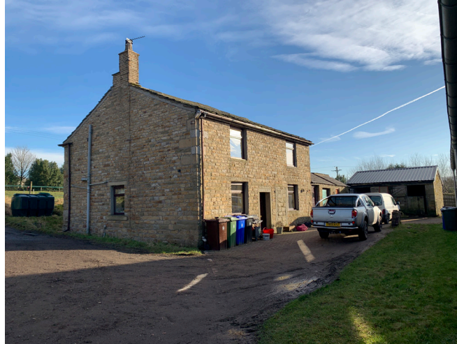
Image 4 - Dry Gap Farmhouse Facing Dry Gap Barn
