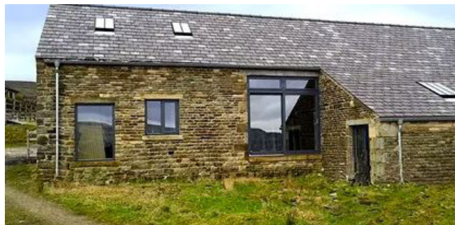
Image 3 - Dry Gap Barn west elevation post conversion
