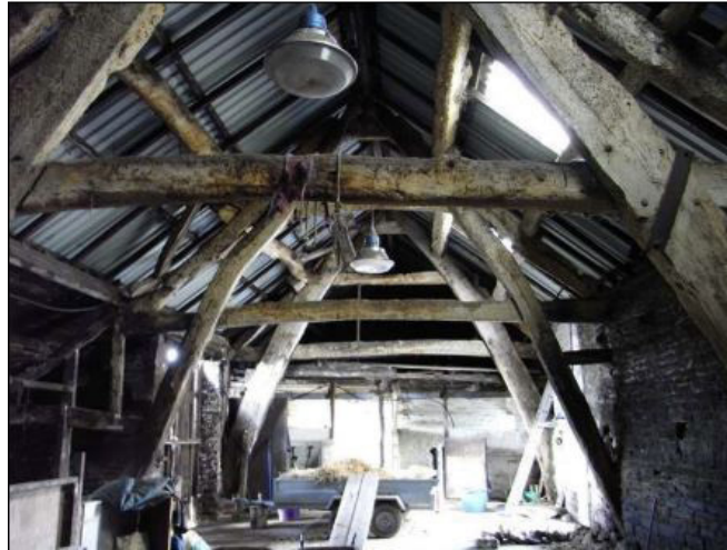
Image 1 - Dry Gap Barn A Frame Structure pre conversion
