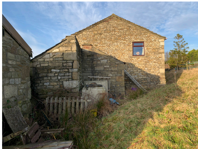
Image 3 - Dry Gap Farmhouse south elevation - lean to structures for removal
