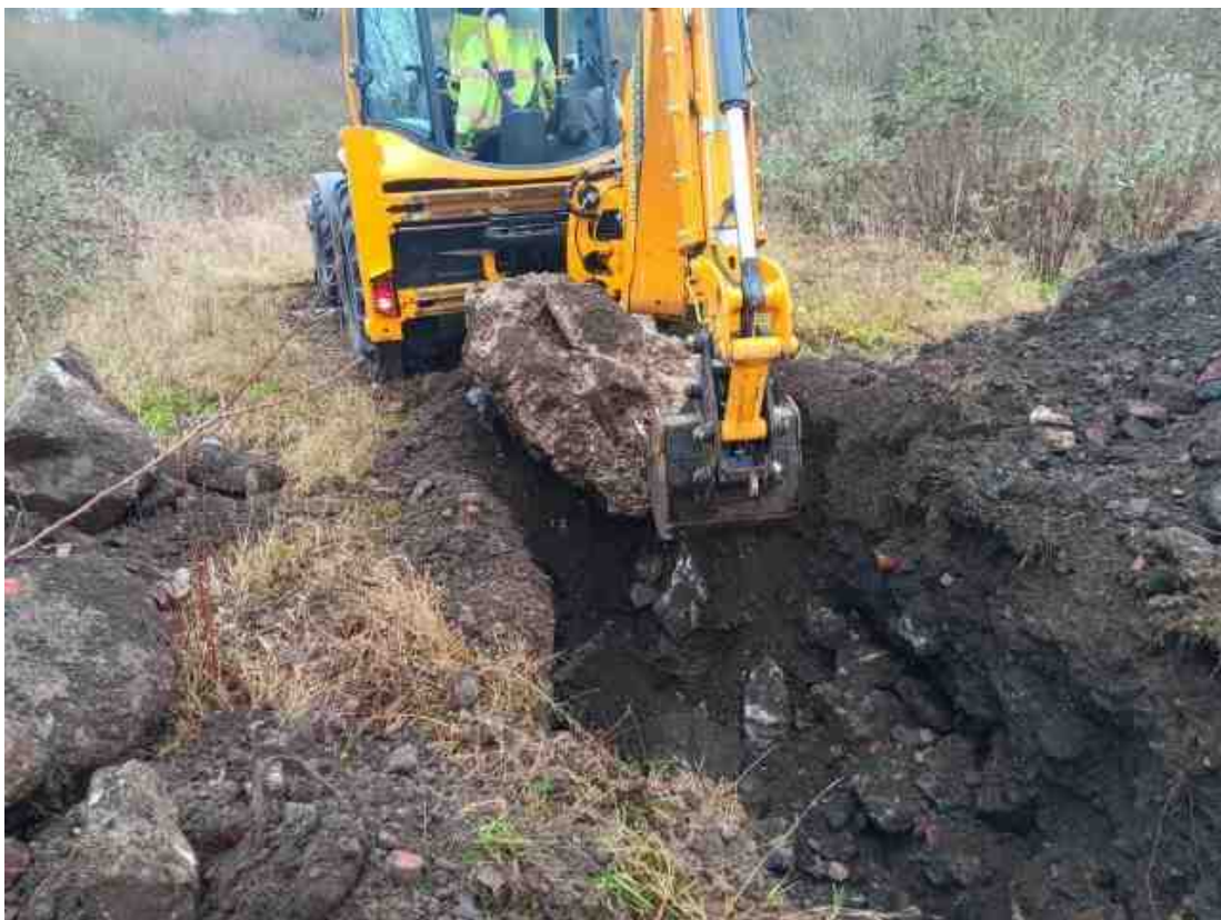
Plate 5-1: Large boulders encountered during the trial pitting.
