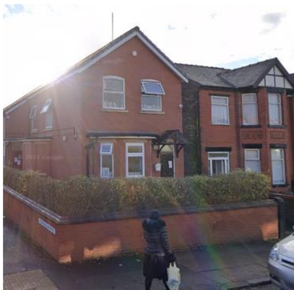
Figure 1 Street view of site (left) and neighbouring property
