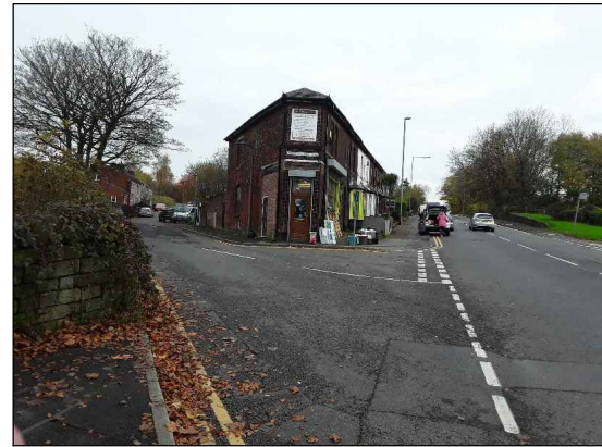
Corner of Woodgate Hill Rd & Rochdale Rd..
