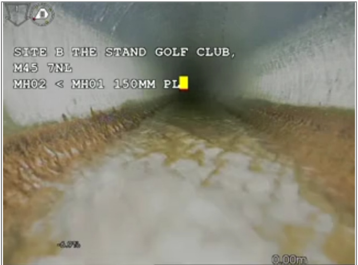
Water level 10% height/diameter
