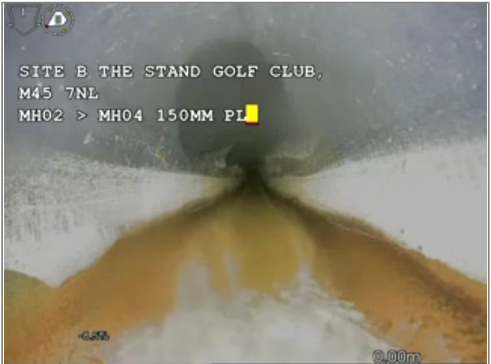
Water level 10% height/diameter
