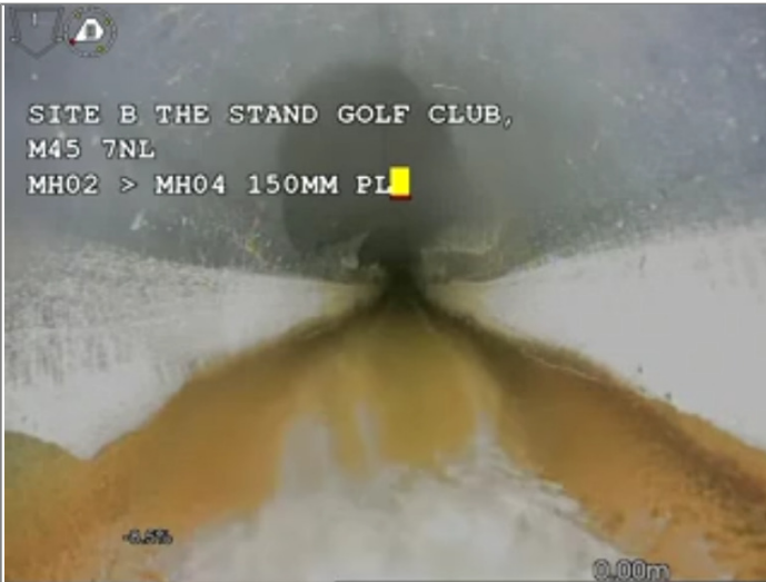
Start node type, Manhole, reference MH02
