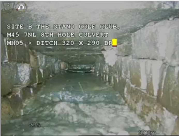
Start node type, Manhole, reference MH05
