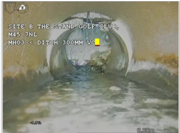
Water level 10% height/diameter
