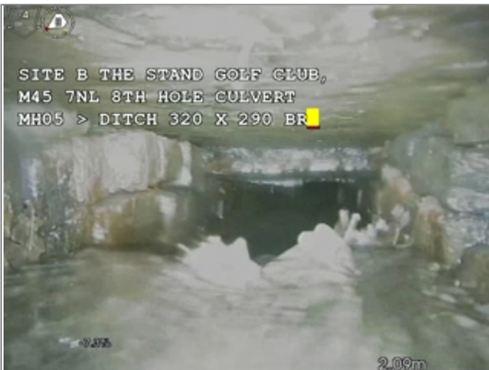
Survey abandoned - Remark: SA due to step down within culvert, unable to pass
