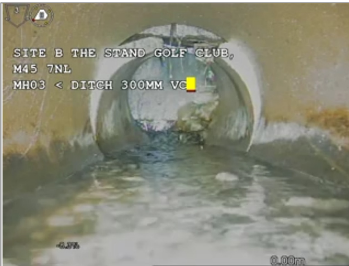
Start node type, Manhole, reference MH03
