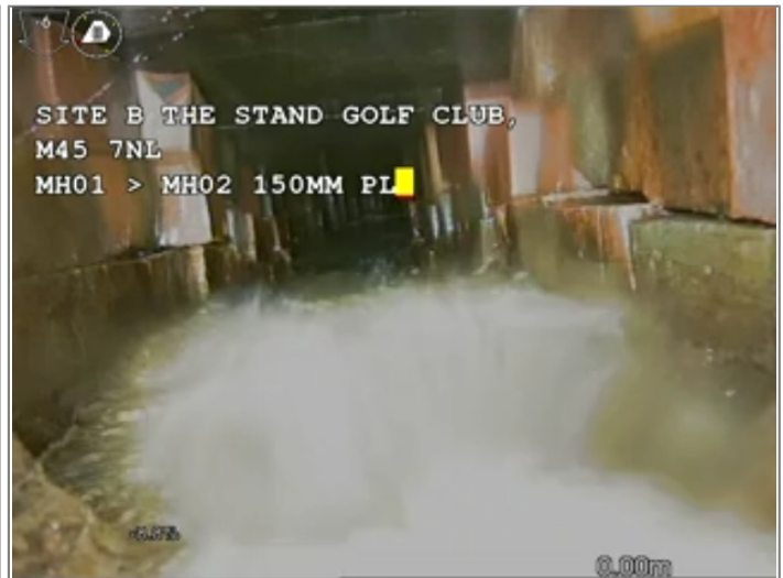
Water level 10% height/diameter
