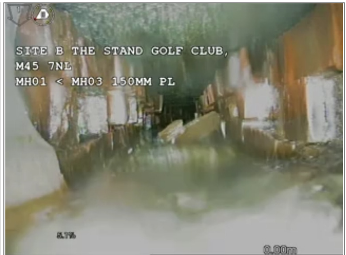
Water level 10% height/diameter
