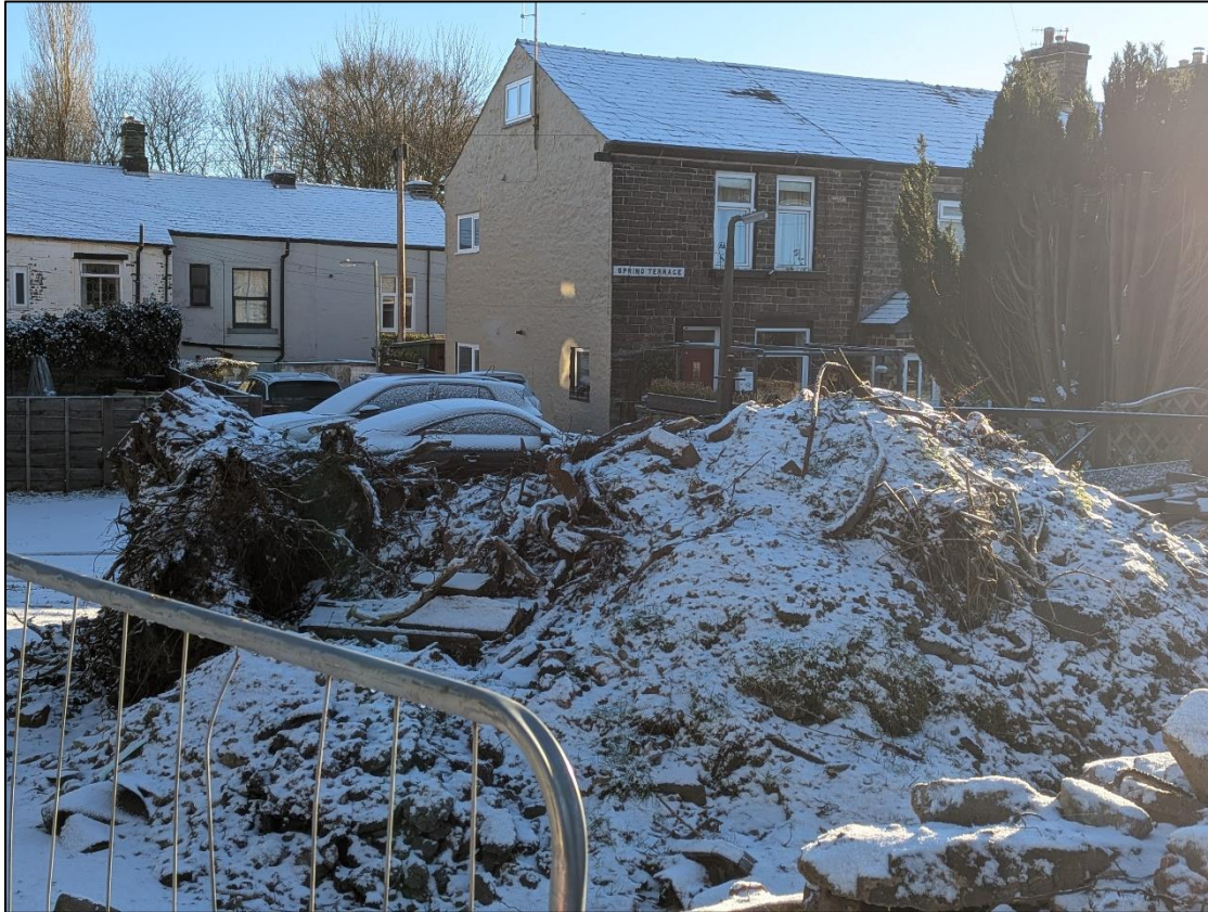
Plate 3: View of the site to the southeast
