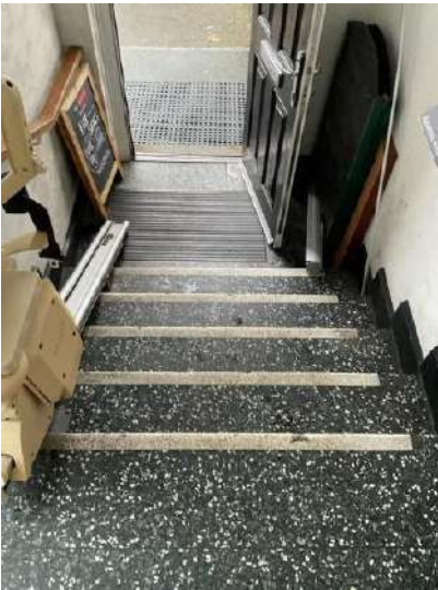
Fig.29 Poor accessibility [ Drees & Sommer]
