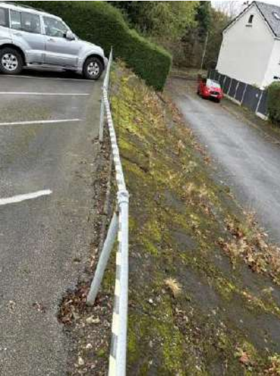
Fig.31 Poor parking [ Drees & Sommer]
