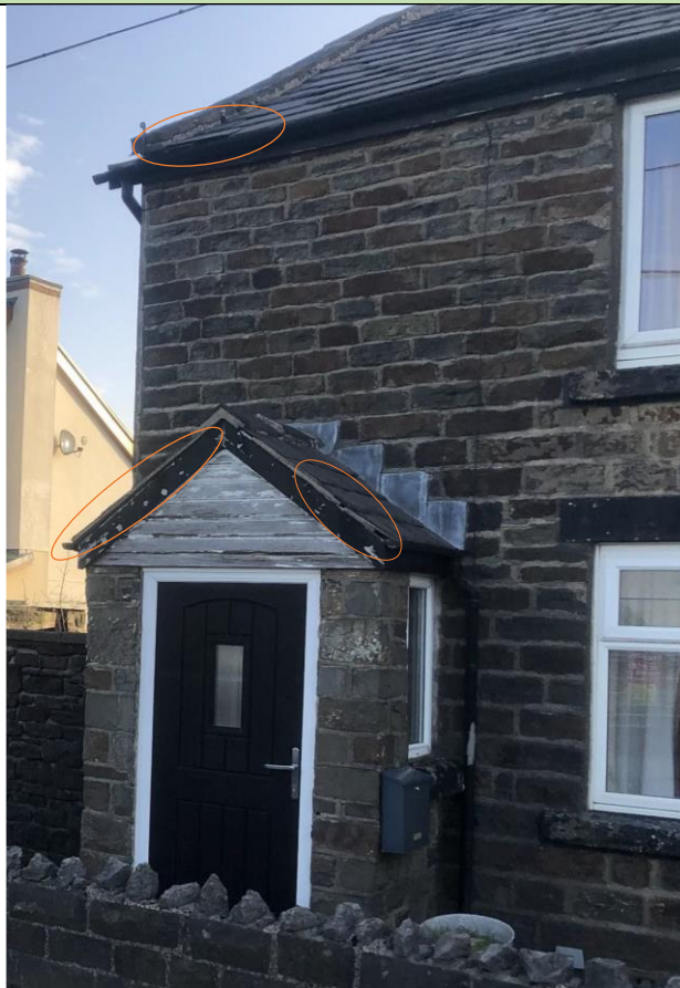
Plate 3: Gaps inspected at front of property
