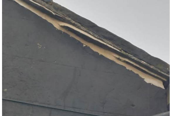
Plate 2: Sealed tiles on gable end.
