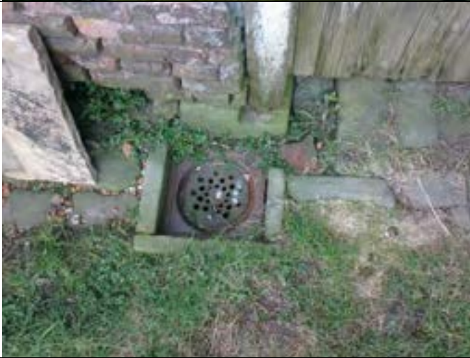
Photograph 8: Drain for the building to the north west of the site.
