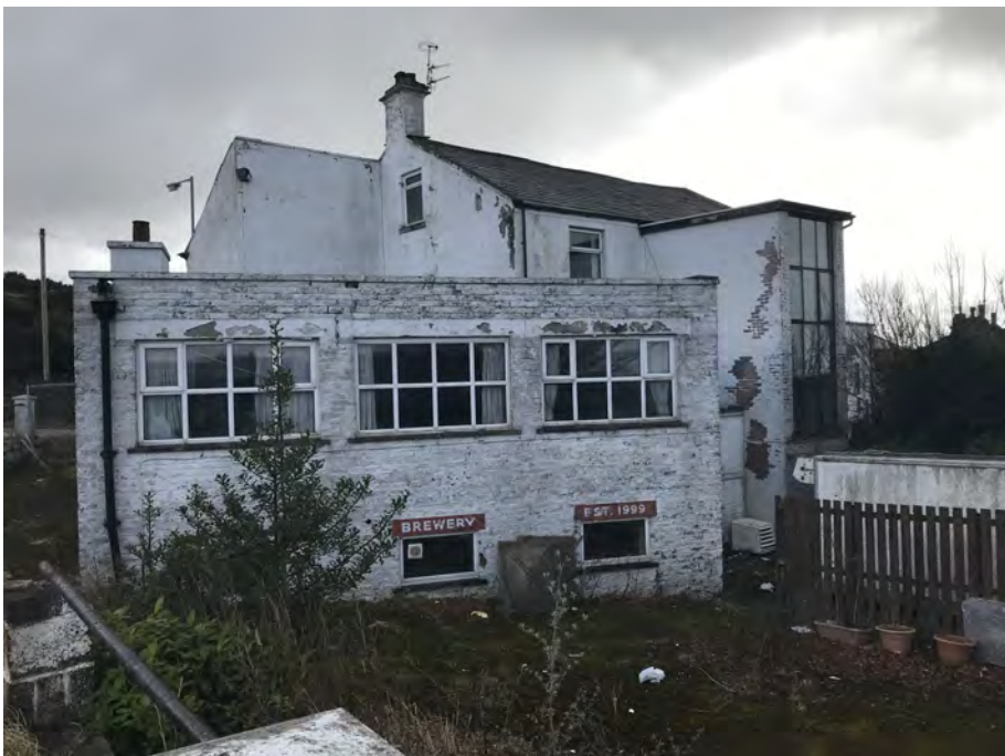
Figure 16: Western (rear) elevation of Lord Raglan Public House
