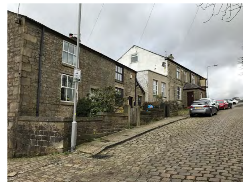
Figure 4: View looking north on Walmersley Old Road
