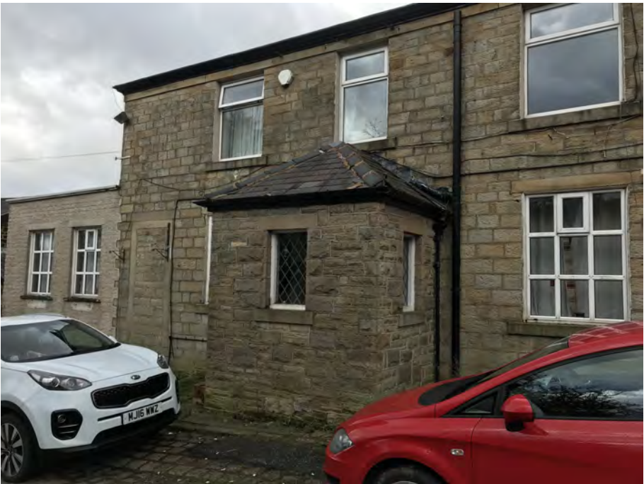
Figure 14: Eastern (front) elevation of Lord Raglan Public House showing porch and flat-roofed extension to the south.
