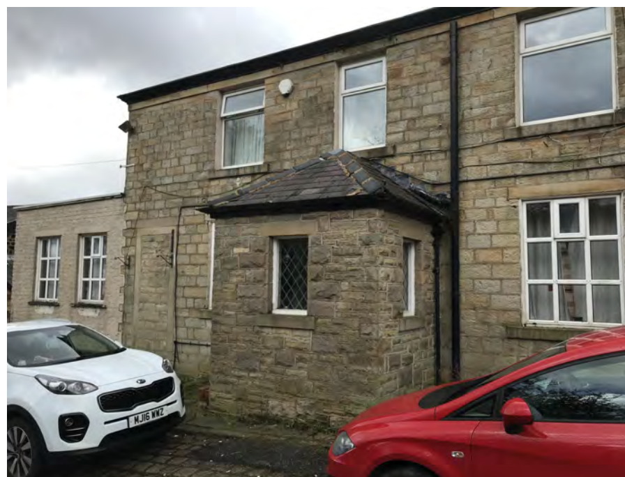
Figure 1: Eastern (front) elevation of Lord Raglan Public House
