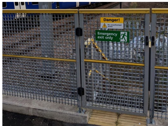
G01 - Maintenance Gate
