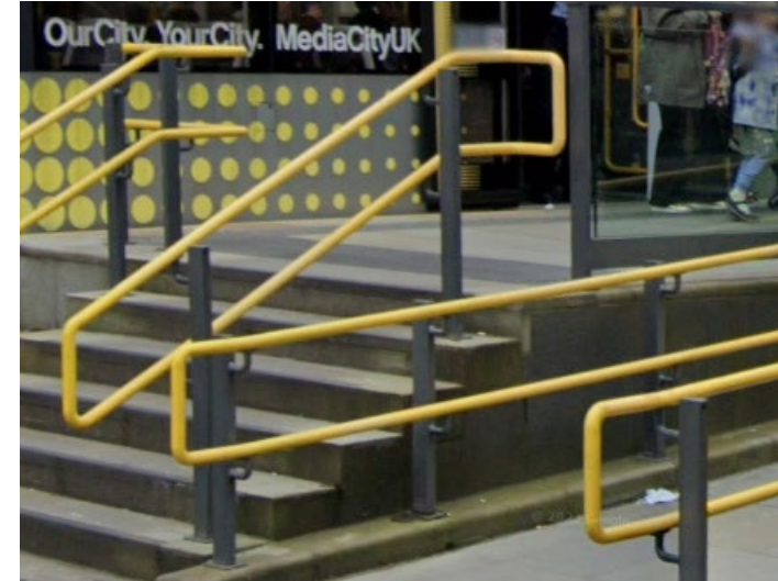
H01 - Steel Handrail
