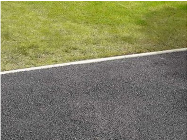
K03 - Kerb Type 3 Pin kerb Supplier: Marshalls
