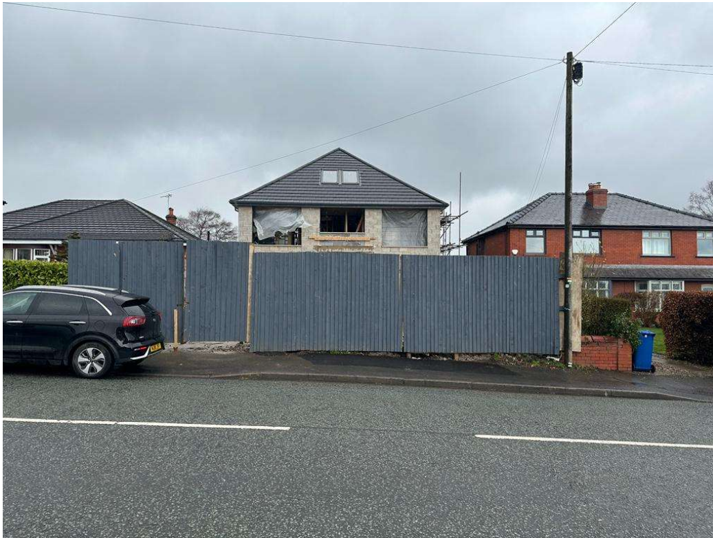
View Point 3. Appeal dwelling , direct view from opposite side of the road
