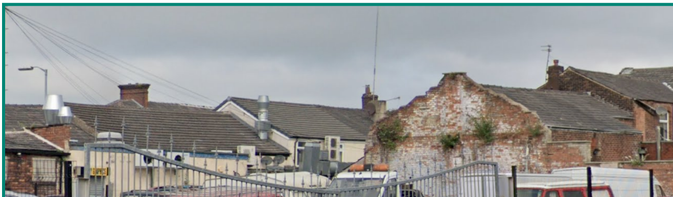
Google Street view showing existing large flues in the street scene as well as a host of extraction units, industrial/commercial metal fencing and a somewhat unkempt gable.
