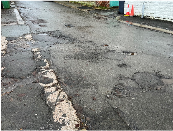
View 8 Spring Street road surface
