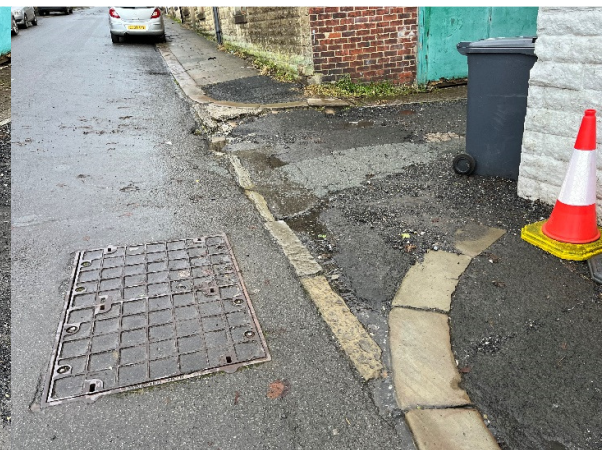
View 13 Caltha Street right side junction
