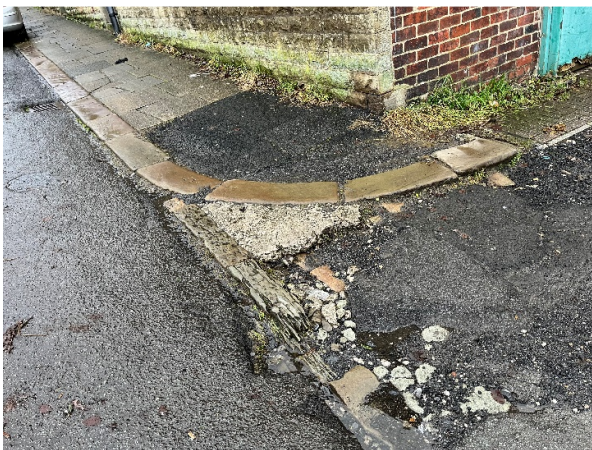
View 12 Caltha Street left side junction
