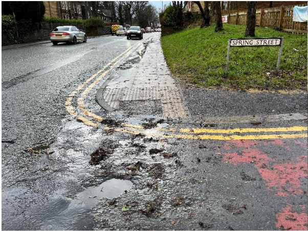
View 2 Pavement at junction with Bolton Street
