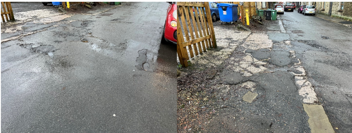
View 6 Spring Street road surface
