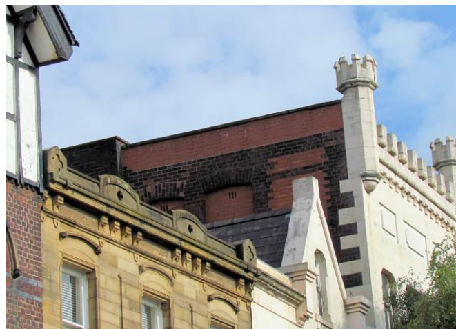
Infilled Windows on Side Elevation
