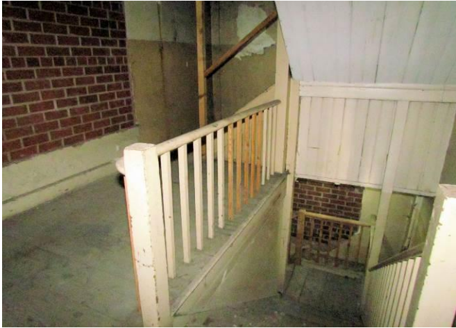
Staircase at North End
