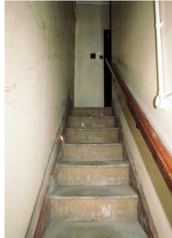
Staircase at South End
