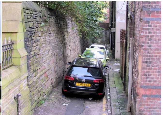
View Along North Back Rock
