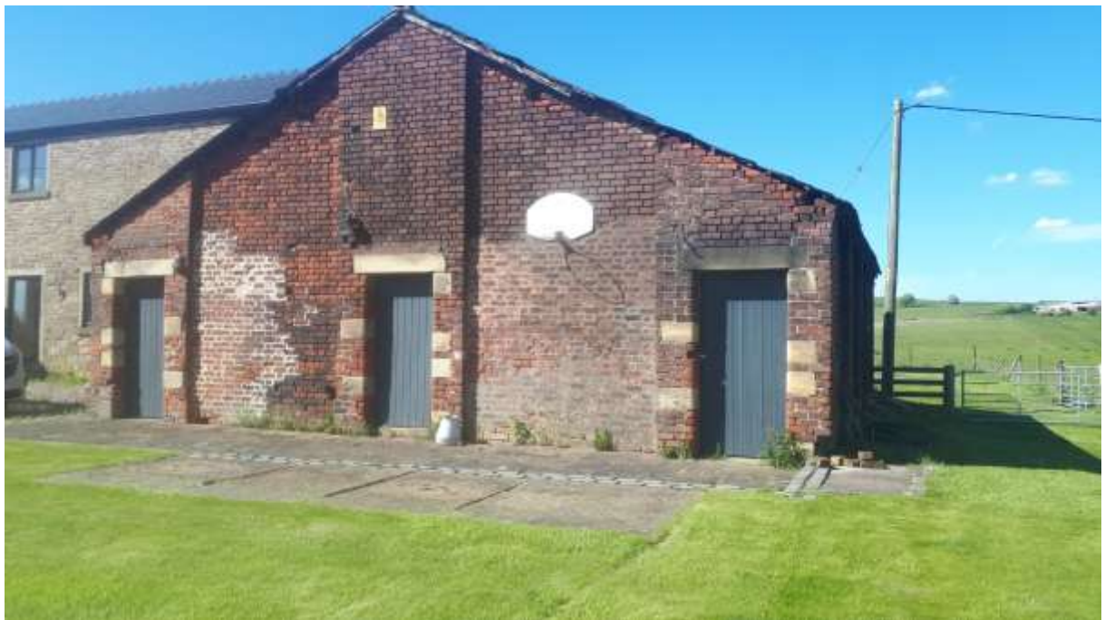
Image 2 – Front elevation of brick shippon (proposed unit 1)
