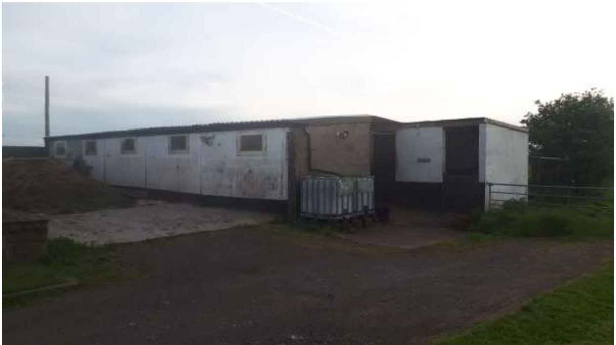
Image 10 – View to front elevation of stables (proposed unit 6)
