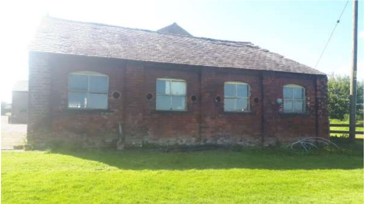
Image 3 – Side/east elevation of brick shippon (proposed unit 1)
