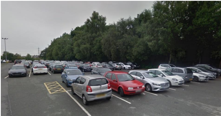
The existing Prestwich Car Park is covered by a surface layer of tarmac
