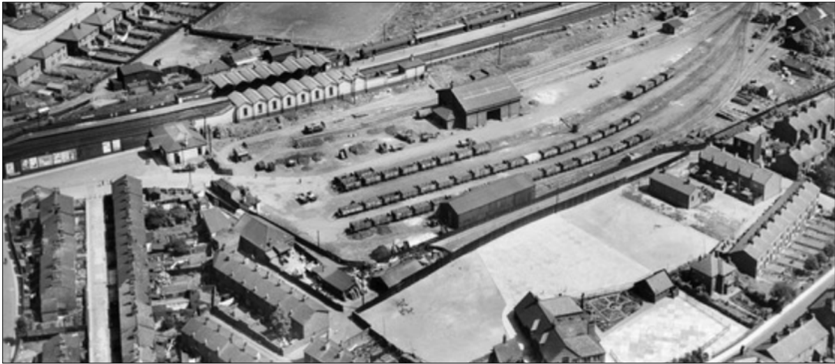
Plate 7 Aerial photograph of Prestwich Railway Station, showing the south of the Site, 1935. Courtesy of Britainfromabove.org.uk
