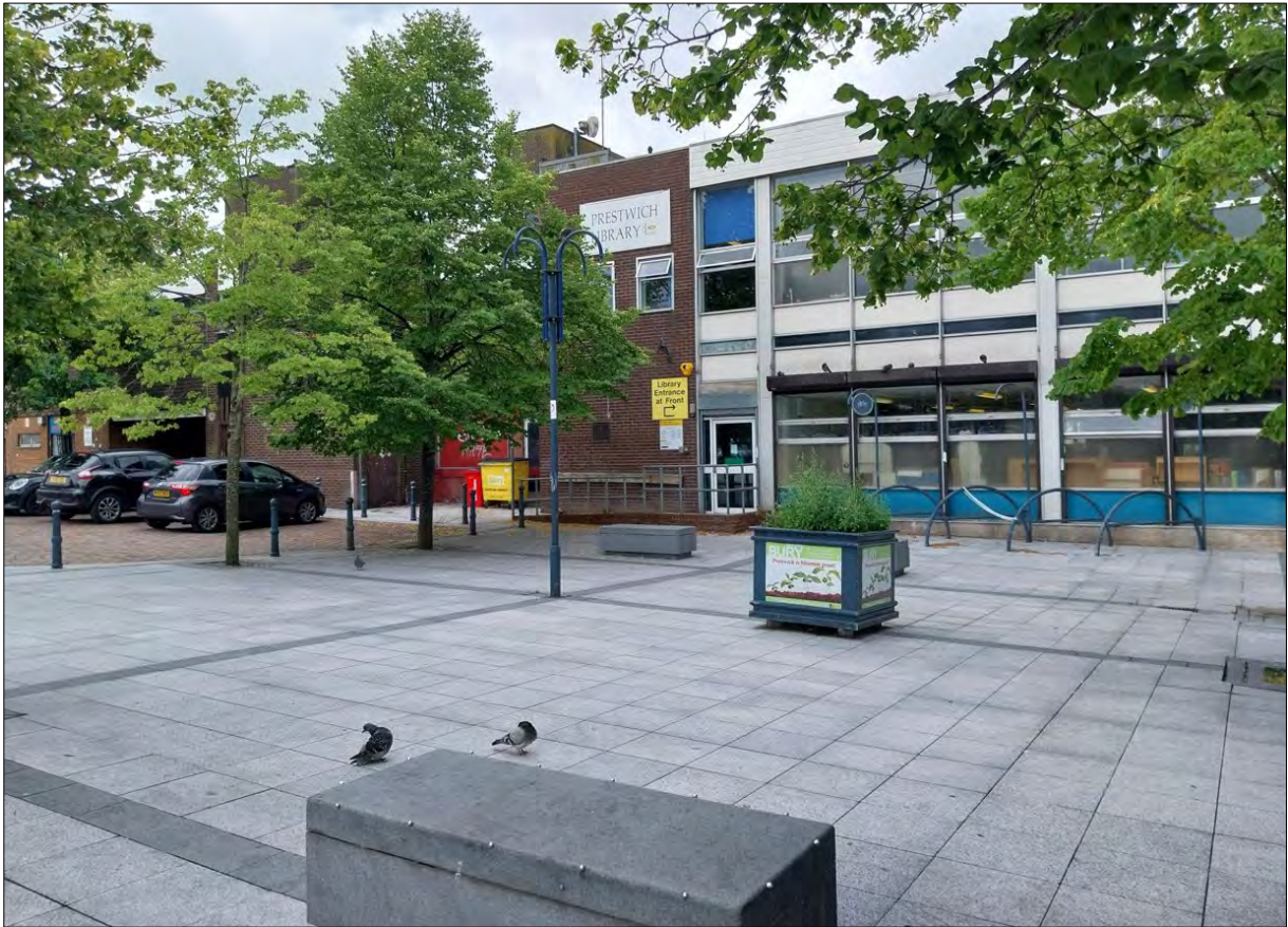
Plate 13 Photograph of the library, facing west
