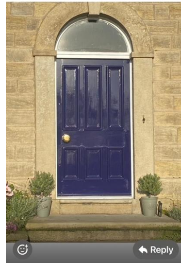
Figure 2. Panelled entrance set beneath a semicircular fanlight. Location: Plant House (next Door)
