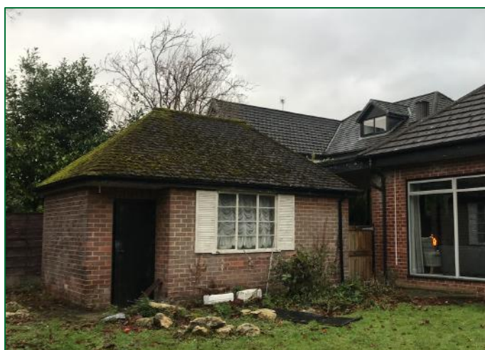
The northeast and southeast elevation of the garage
