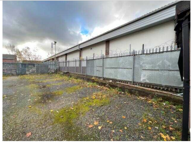
6. Site boundary facing south-west, with rear of Aldi store in background
