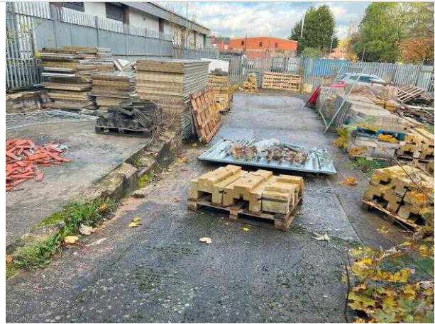
2. Construction material storage – southern half of Site
