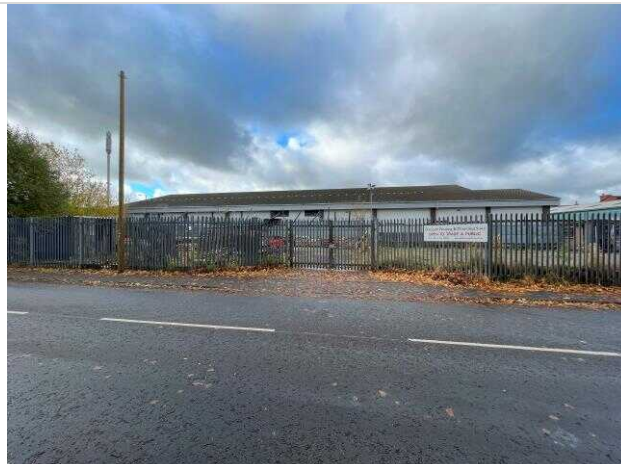
10. View of Site entrance from Huntley Mount Road
