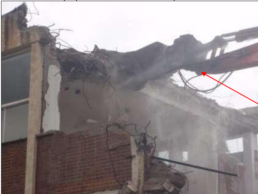
Dust suppression at source
