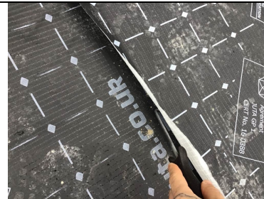
Testing of taped membrane joint
