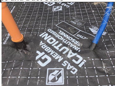
Unit 2 sealed pipe penetrations using SAGM and heat applied
