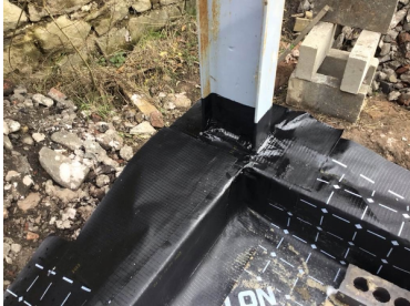
Unit 1 sealed corner detailing using SAGM and heat applied
