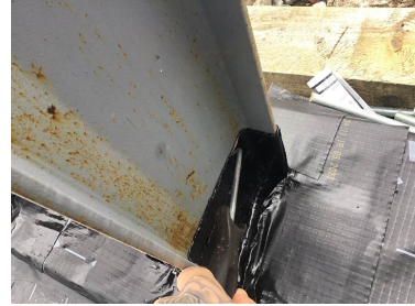
Testing to stanchion detailing
