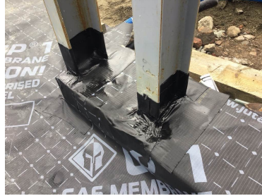
Unit 1 sealed stanchion detailing using SAGM and heat applied
