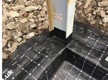
Unit 2 sealed corner detailing using SAGM and heat applied
