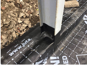
Unit 2 sealed stanchion detailing using SAGM and heat applied
