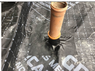
Unit 1 sealed pipe penetration using SAGM and heat applied
