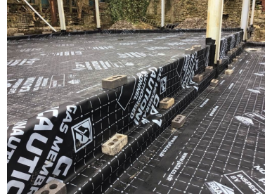
Step down detailing using Juta GP1 membrane
