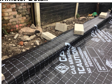
Membrane extended over the perimeter edge blockwork
