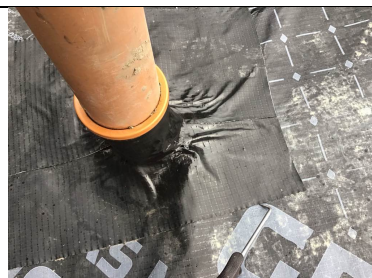
Testing to pipe detailing
