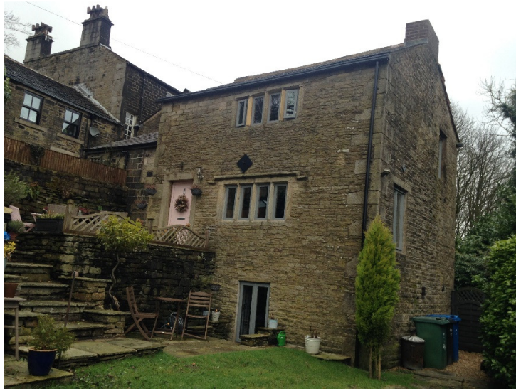
3 Alba Street looking towards the lower patio
